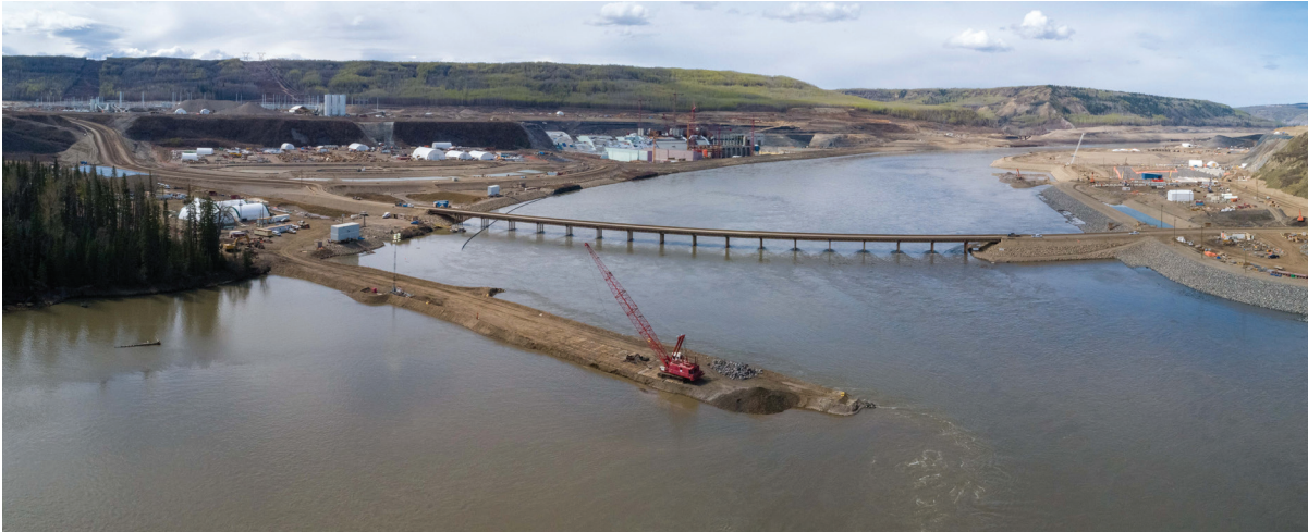
Construction of the Site C dam across the Peace River.
