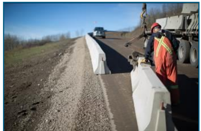
Concrete roadside barrier placement on Old Fort Road south of the realignment
