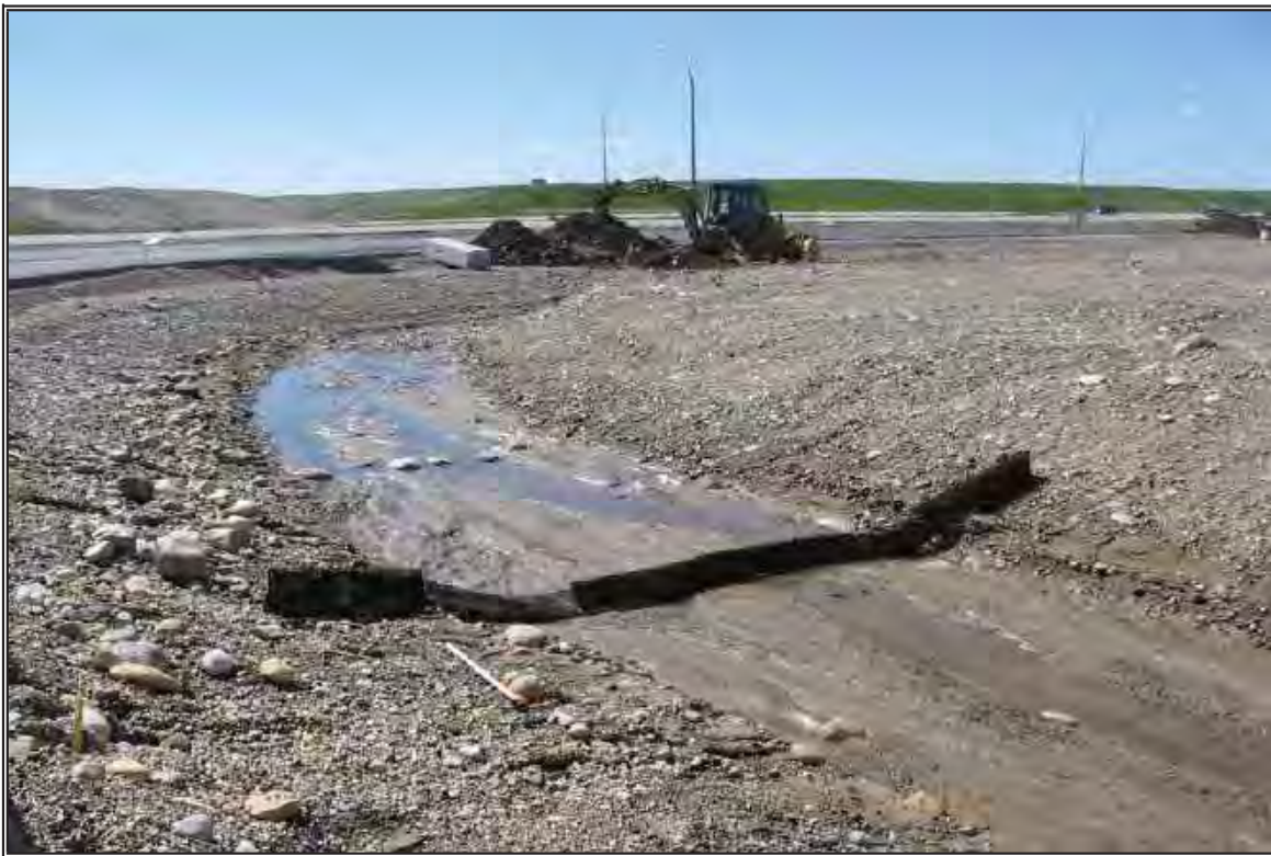
Ditch checks can be subject to washout and undermining if not properly installed (spacing, anchoring, and configuration) or used as part of a system of erosion & sediment controls.
