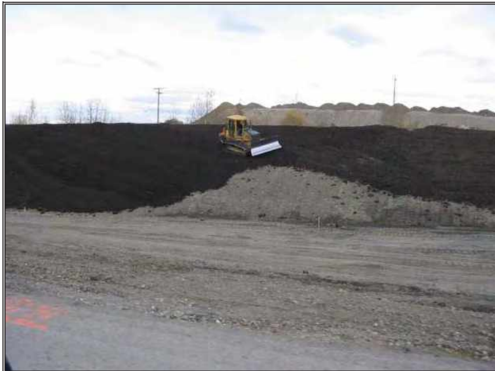
Photo 10: Timely final grading and site preparation, followed by application of topsoil reduces the exposure of highly erodible subsoil to erosion. Upon completion of topsoil application, additional erosion control measures detailed in the Erosion & Sediment Control Plan should be implemented.
