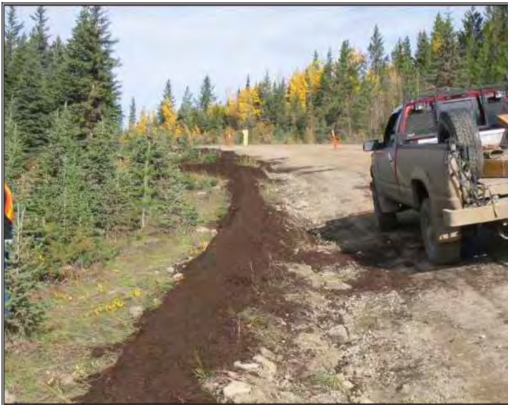
Installation of a compost berm
