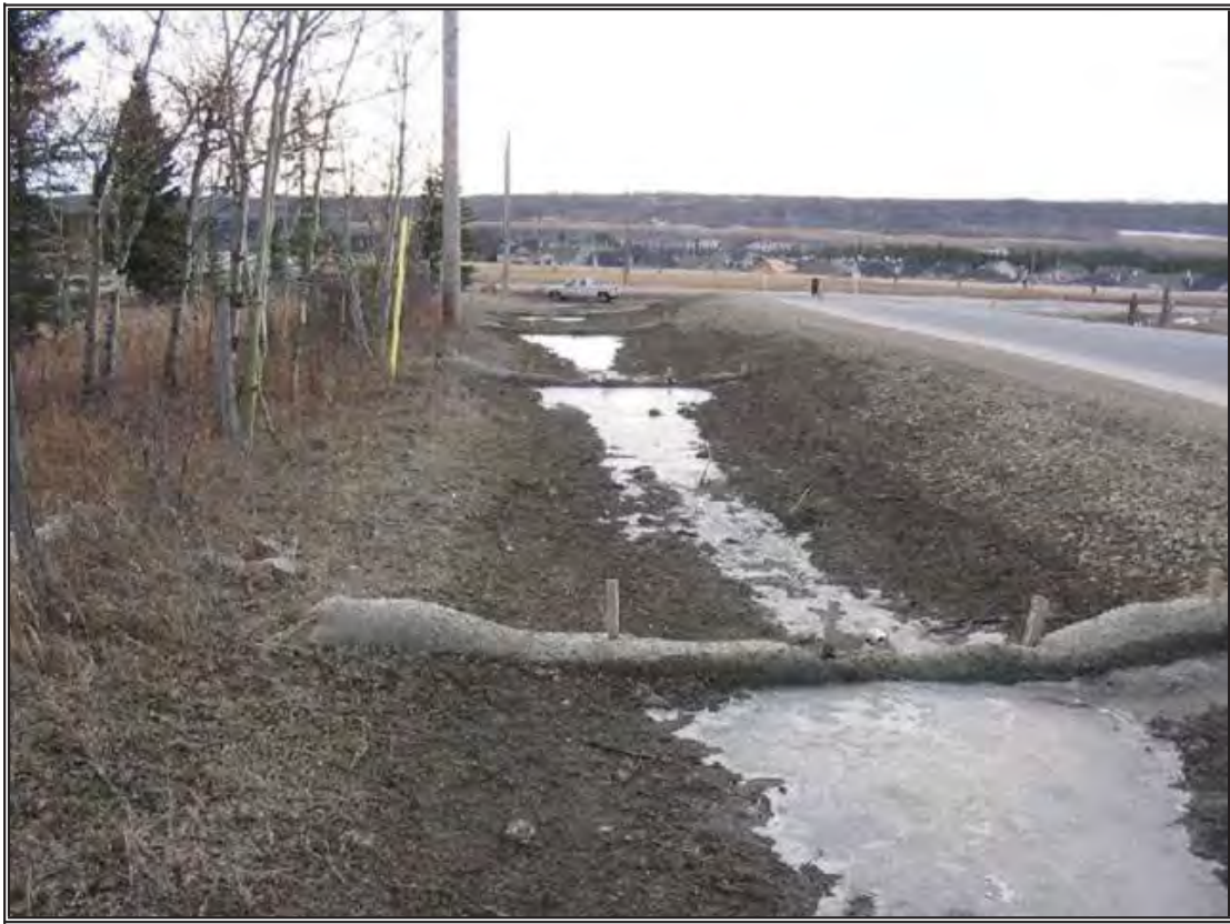
Straw wattles provide an excellent type of ditch check in small ditches conveying small volumes of run-off.
