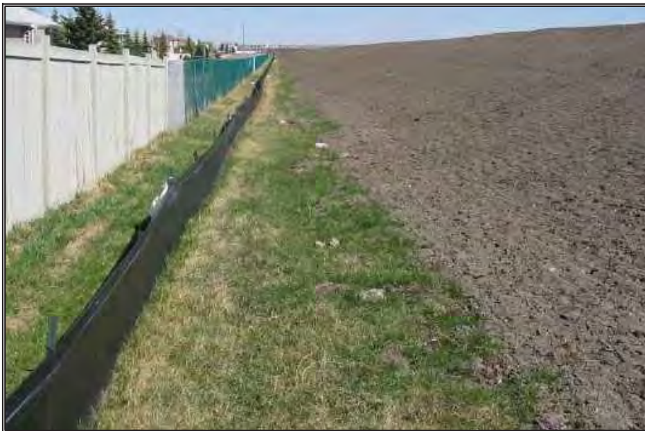
Use of a vegetated buffer strip in combination with a perimeter silt fence and a topsoiled and tracked slope. BMPs work most effectively if they are implemented as part of a system of erosion & sediment control.
