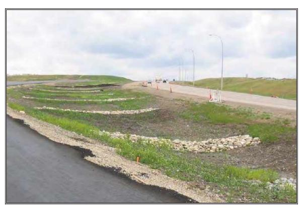
A system of well-installed rock check dams (properly spaced and extended up the sides of the channel) on a road construction project.
