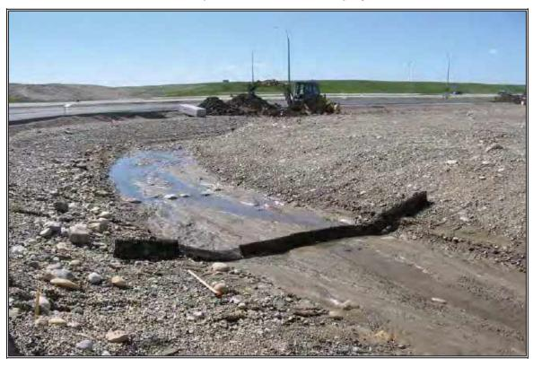
Ditch checks can be subject to washout and undermining if not properly installed (spacing, anchoring, and configuration) or used as part of a system of erosion & sediment controls.
