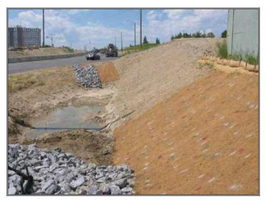
Simple sediment trap, with stabilized inlet and outlet and application of an erosion control blanket to protect side slopes.
