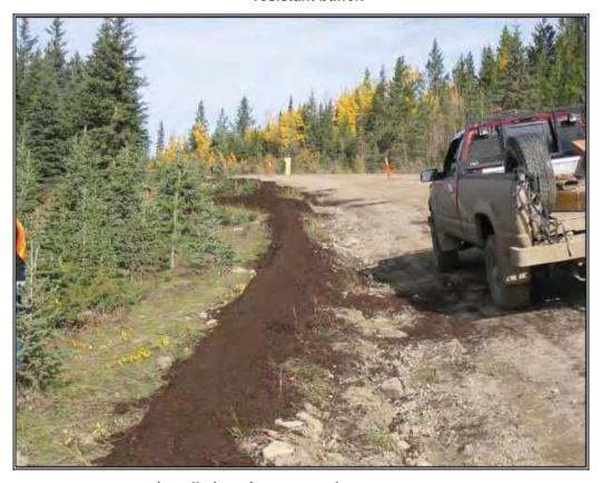
Installation of a compost berm
