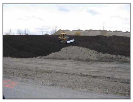
Photo 10: Timely final grading and site preparation, followed by application of topsoil reduces the exposure of highly erodible subsoil to erosion. Upon completion of topsoil application, additional erosion control measures detailed in the Erosion & Sediment Control Plan should be implemented.
