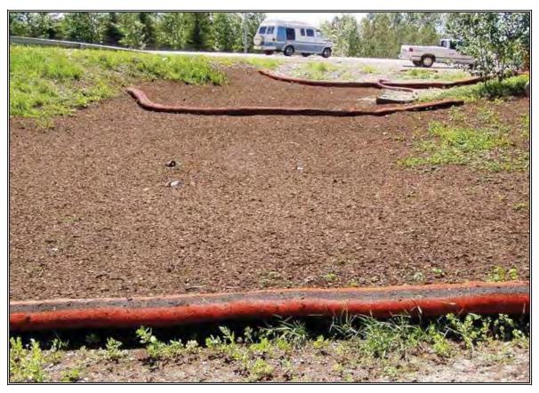
Photo 21: Combination of compost socks and a compost blanket applied to control erosion adjacent to a sensitive creek. A design seed mix was incorporated with the application, resulting in long-term erosion control. Biodegradable compost sock liners are also available.
