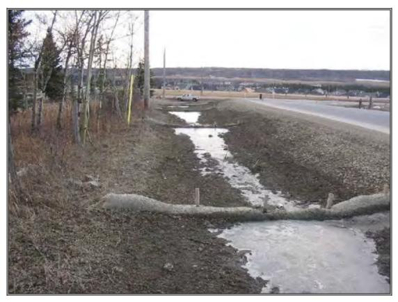
Straw wattles provide an excellent type of ditch check in small ditches conveying small volumes of run-off.
