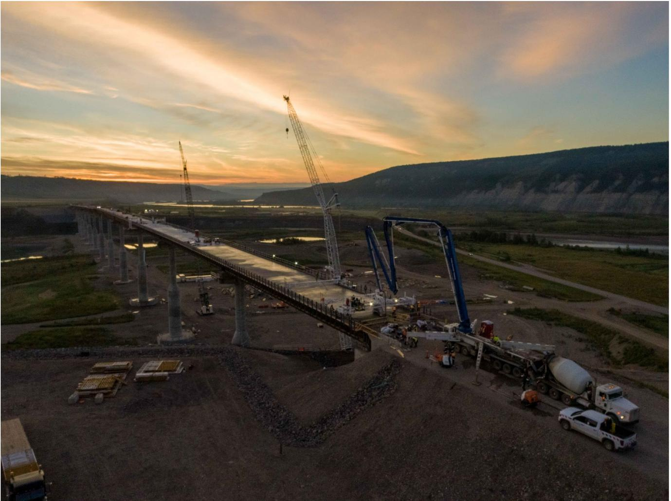
Crews completed the final concrete deck pour on the Halfway River bridge segment of Highway 29 recently. About 200 trucks' worth of concrete was placed on the one-kilometre bridge deck in 13 pours.
