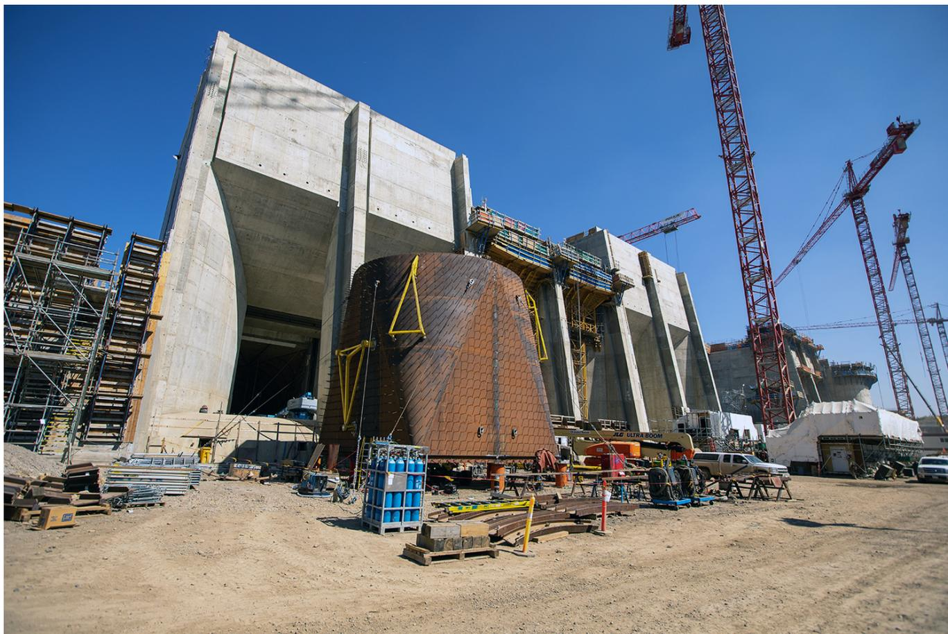
Intake units 1 and 3 are substantially complete, with unit 2 under construction. The unit 4 penstock transition piece is pictured in the foreground. See more project photos in the [image gallery](#).
