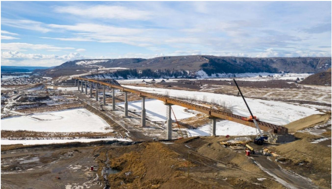
Crews completed installing the steel bridge girders – the main horizontal support beams – across the Halfway River bridge. The girders were assembled in 27 sections with 81 separate pieces. See more project photos in the [image gallery](#).
