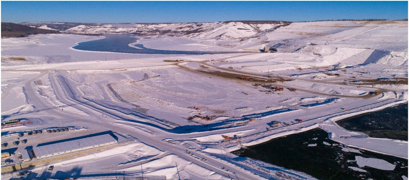
The upstream cofferdam was recently completed to its final elevation, approximately 24 metres high above the riverbed. The upstream and downstream cofferdams seal off the Peace River and direct water through two diversion tunnels. See more project photos in the [image gallery](#).
