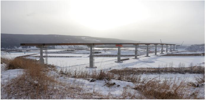
All twelve bridge piers for the Halfway River are now complete and steel girders are being installed on top. In this area, the reservoir will cover the existing highway and bridge, requiring re-alignment of the highway and construction of a new bridge. This new segment of highway will be three kilometres long, and the new bridge will be one kilometre long. See more project photos in the <u>image gallery</u>.
