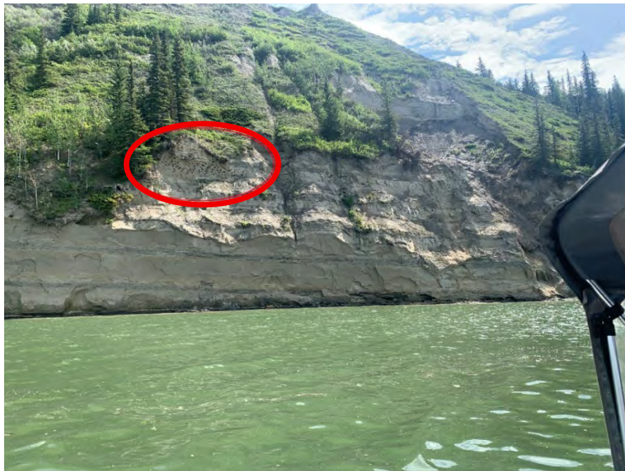
Figure 6: Erosion at the base of an existing colony (red ellipse) in high, eroding slope habitat. Pre-inundation, this colony was well above the reservoir and erosion events were likely less common. Since inundation, the base of this high slope is now underwater, and shoreline erosion is actively removing the supporting material of this colony.
