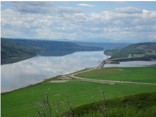
Site C Reservoir at Halfway River Confluence. Photo Credit: Neil Simpson
