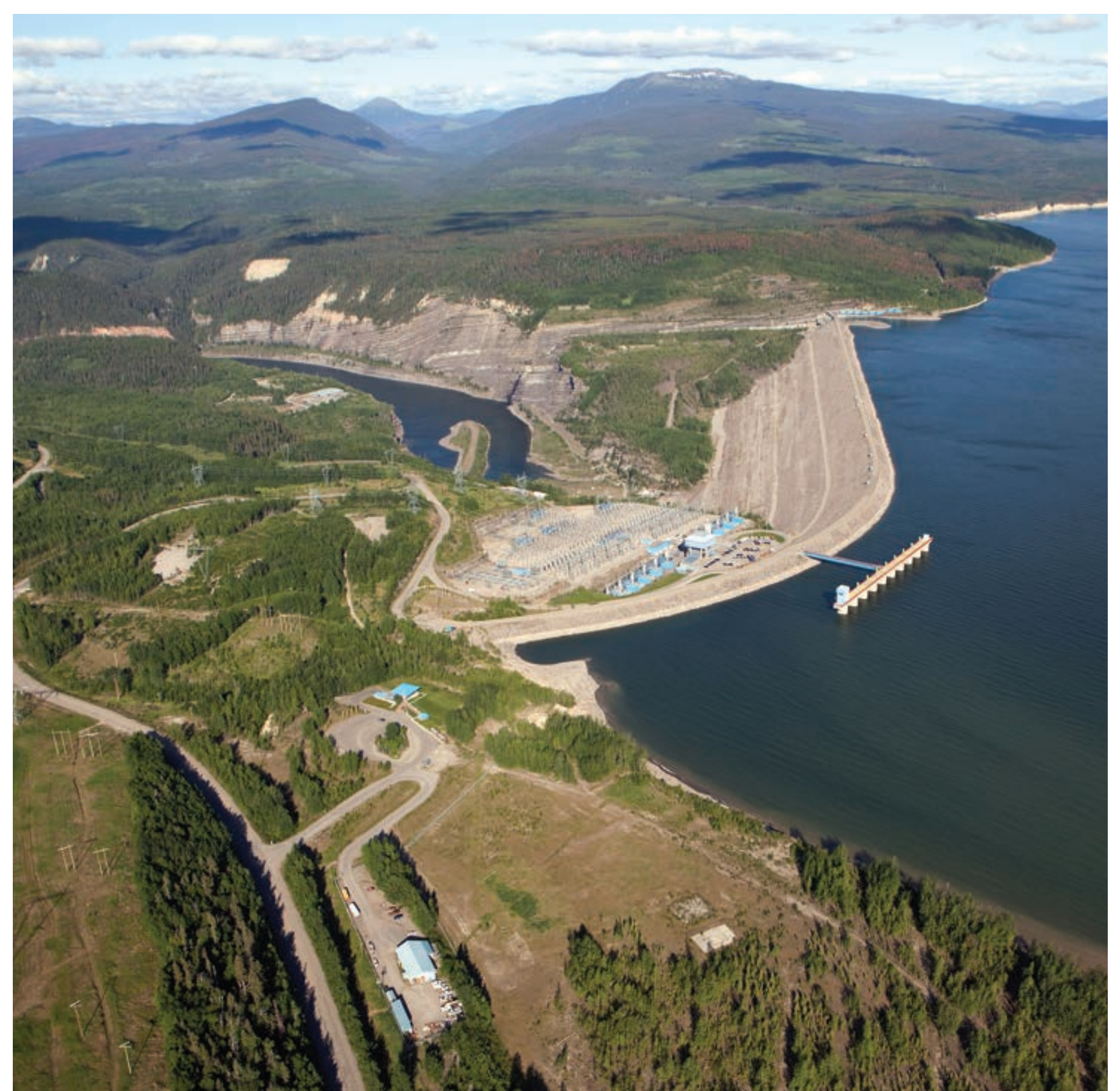
W.A.C. Bennett Dam
