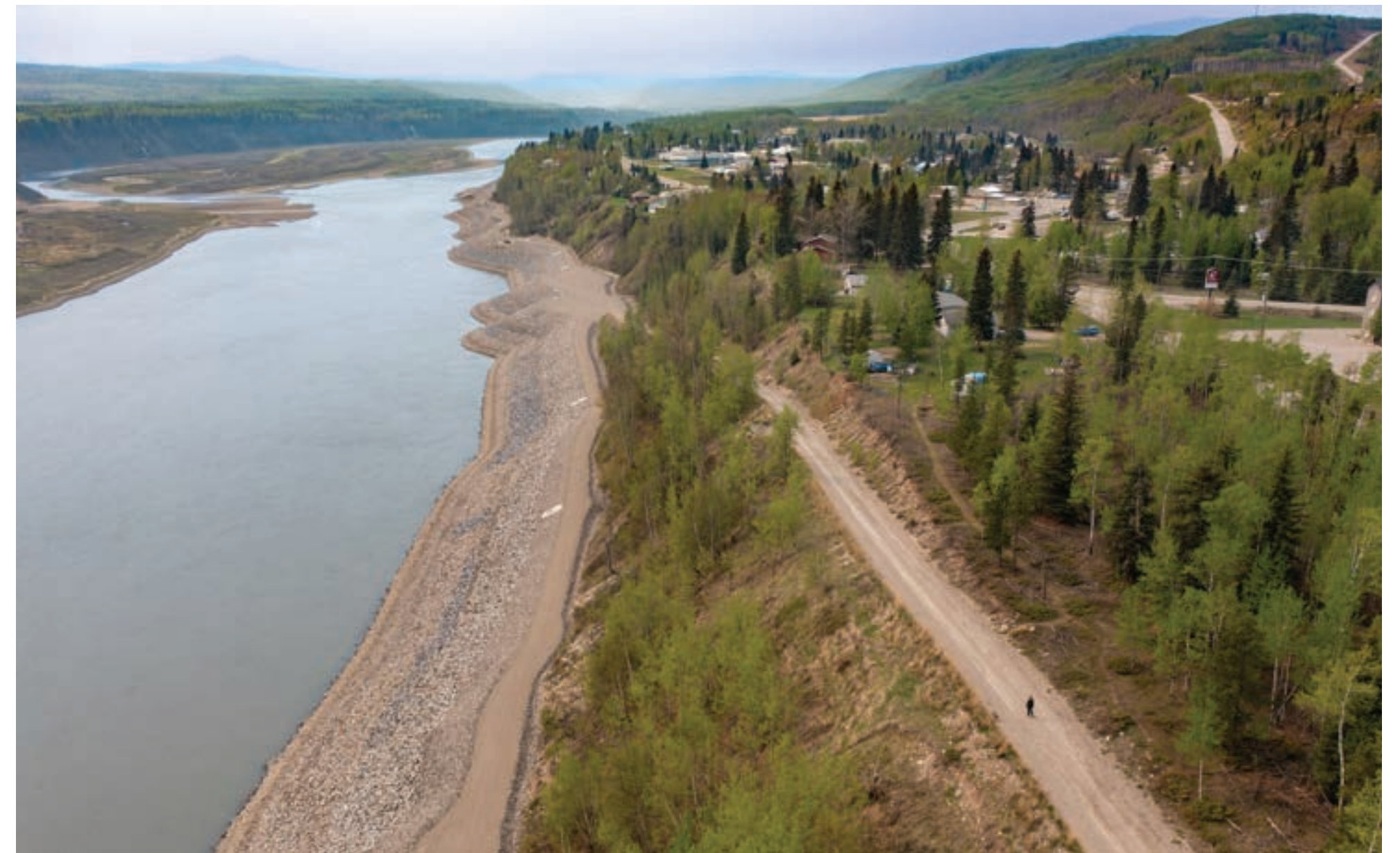
The shoreline protection berm extends for 2.6 km and is made of riprap, rocks and gravel.
