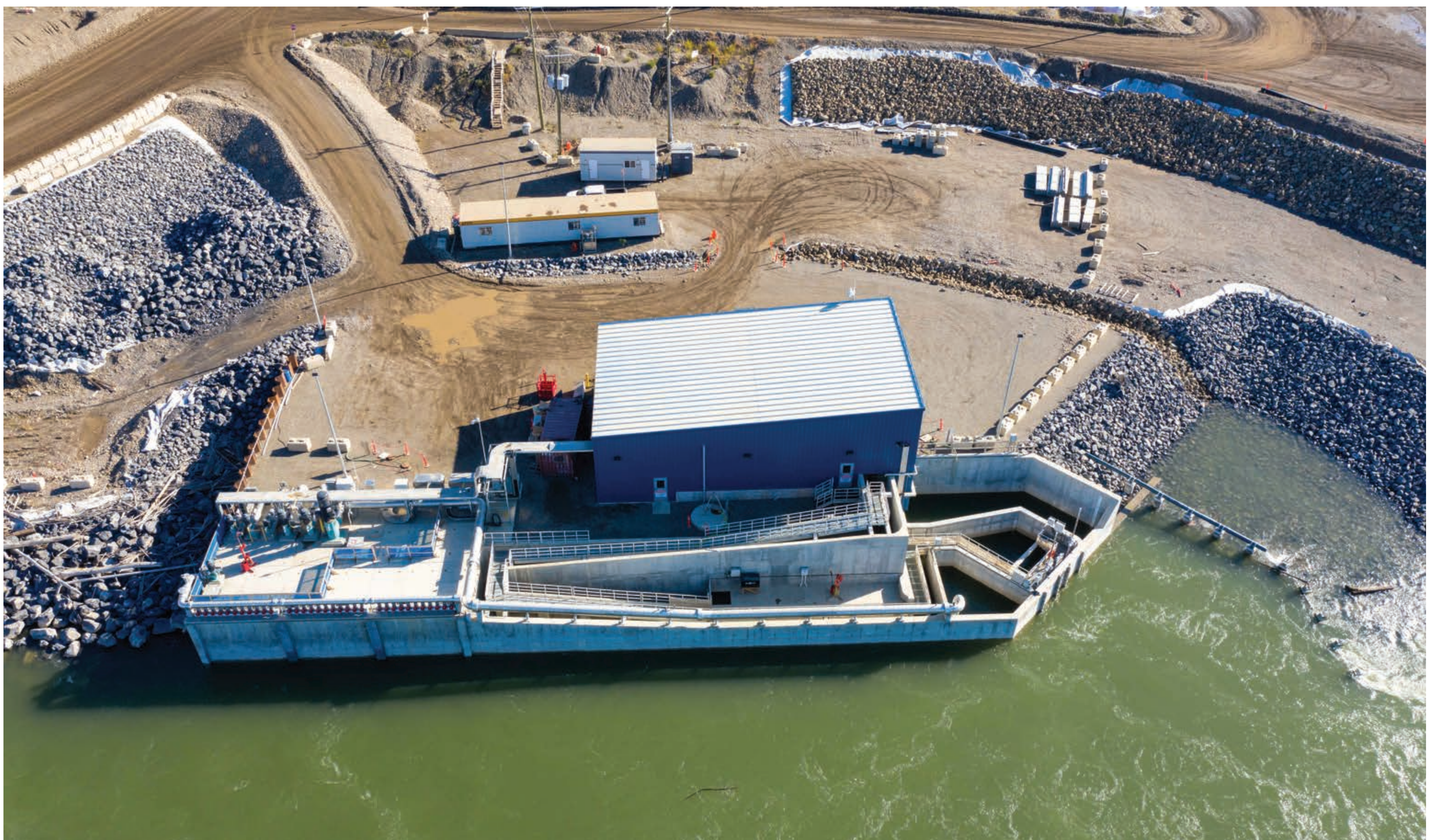
We built a temporary fish passage facility for use during dam construction. We used what we learned from the temporary facility to build the permanent facility.
