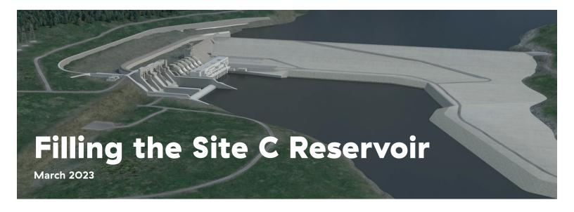
One of the last milestones in building the Site C dam is to fill the reservoir. Filling the reservoir with water allows us to put the generating station, spillways, turbines and generators into operation, creating enough energy to power the equivalent of about 450,000 homes per year in B.C.
