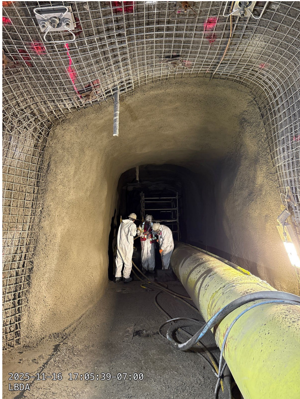
Figure A-9 Left Bank Drainage Adit - Production bolting, mesh and shotcrete placement (November 2025)
