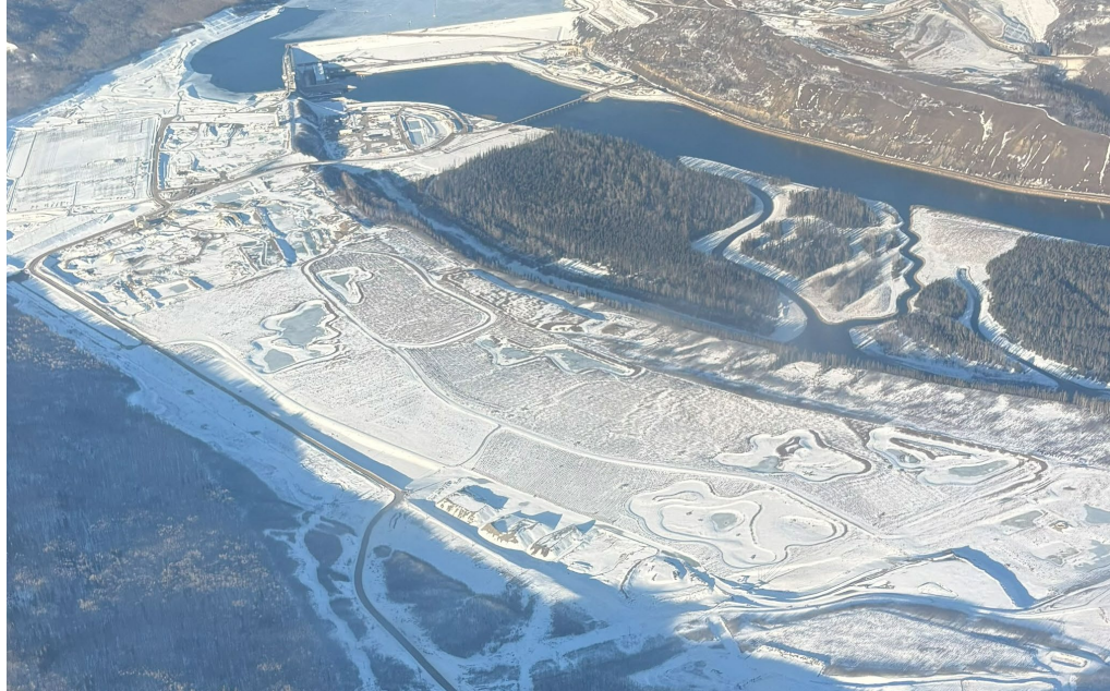
Figure A-18 Area A Reclamation (January 2026)
