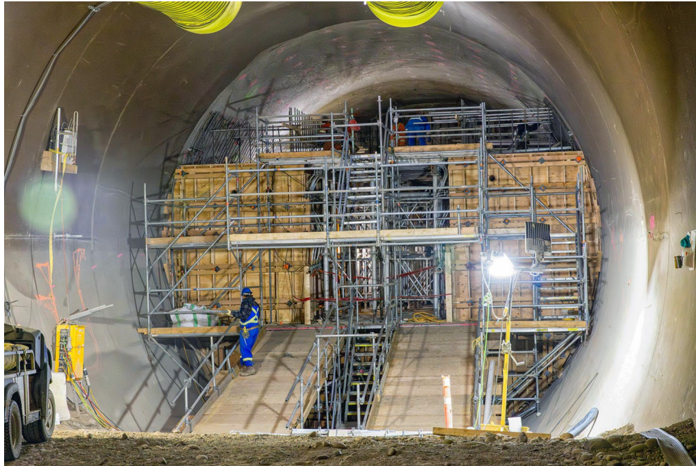
Figure A-10 Construction of the concrete plug for the Diversion Tunnel 1 backfilling (November 2025)
