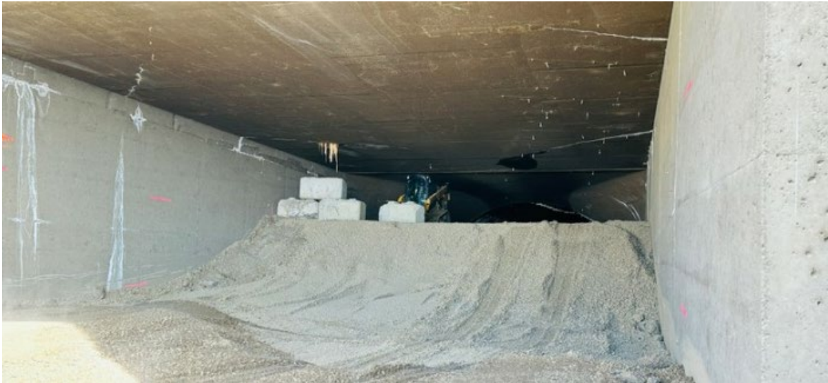
Figure A-28 Diversion Tunnel 1 and 2 Outlet – Setting up Lock Blocks For Backfill (March 2026)
