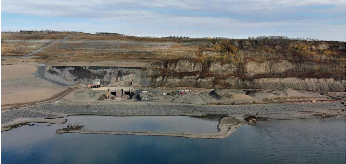
Figure A-5 In-river excavation work. This work will improve fish habitat, reduce fish stranding risk, increase plant discharge capacity and provide gravel for the diversion tunnels. (October 2025)
