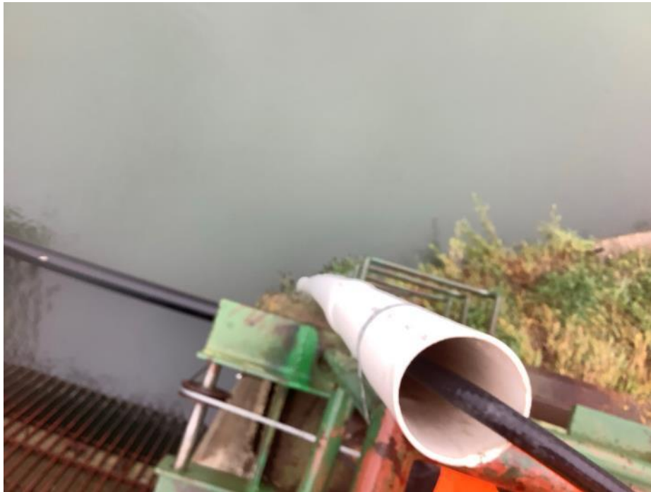
Figure 1. PVC pipe attached to the upstream wingwall of the McMahon Gas Plant intake forebay which contains the Analite turbidity sensor and the TidbiT water temperature sensor.
