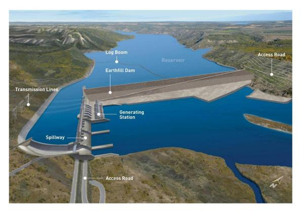
Figure 2.1 General Arrangement of Earthfill Dam and Concrete Structures
