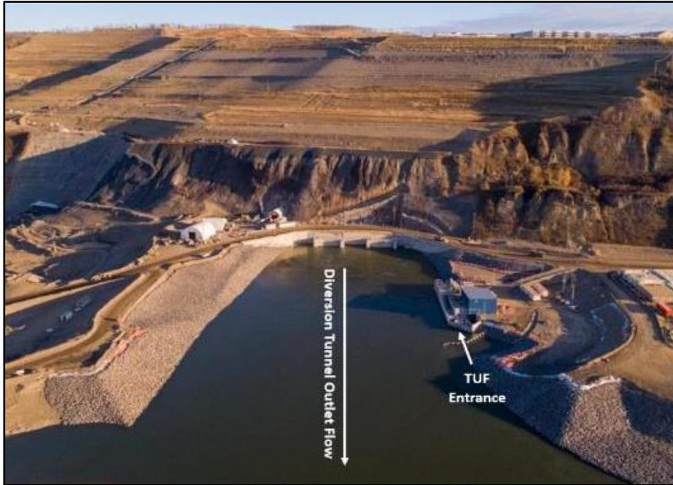
Figure 1. Aerial photo of the temporary upstream fish passage facility (TUF) on the Peace River, diverted through two tunnels which do not allow for upstream fish passage. The TUF is located on the east bank of the diversion tunnel outlet. Photo provided by BC Hydro, June 8, 2021.
