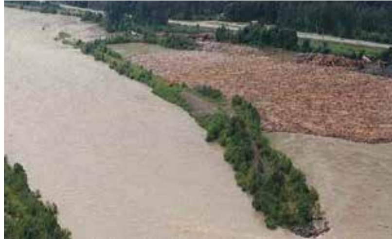
Fraser River debris trap and fin boom
