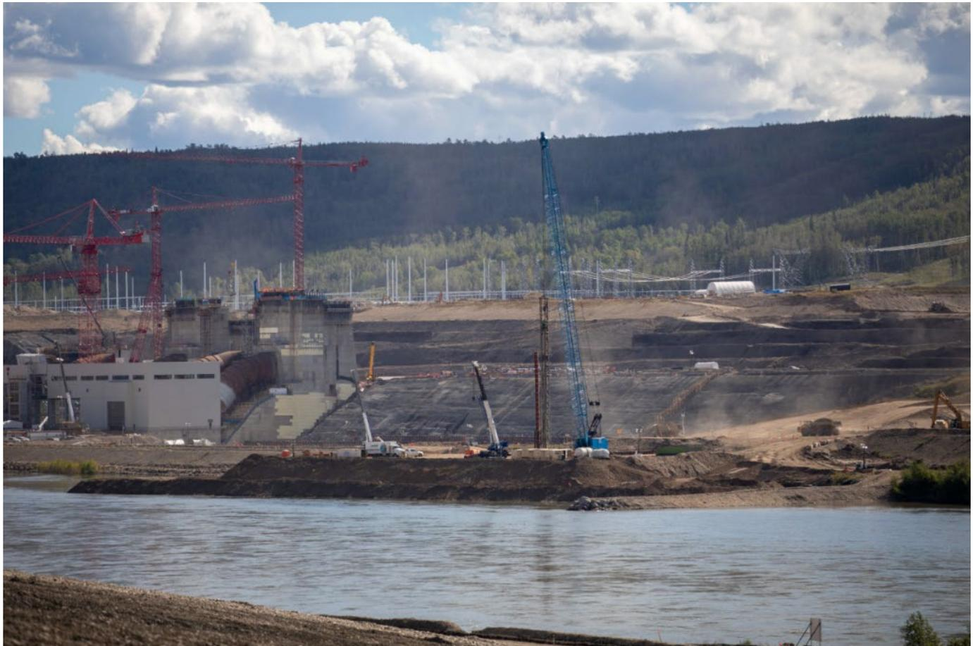
We continue to build the upstream cofferdam across the river. Once fully across, the cofferdam will seal off the river and channel the water into the diversion tunnels. See more project photos in the [image gallery](#).
