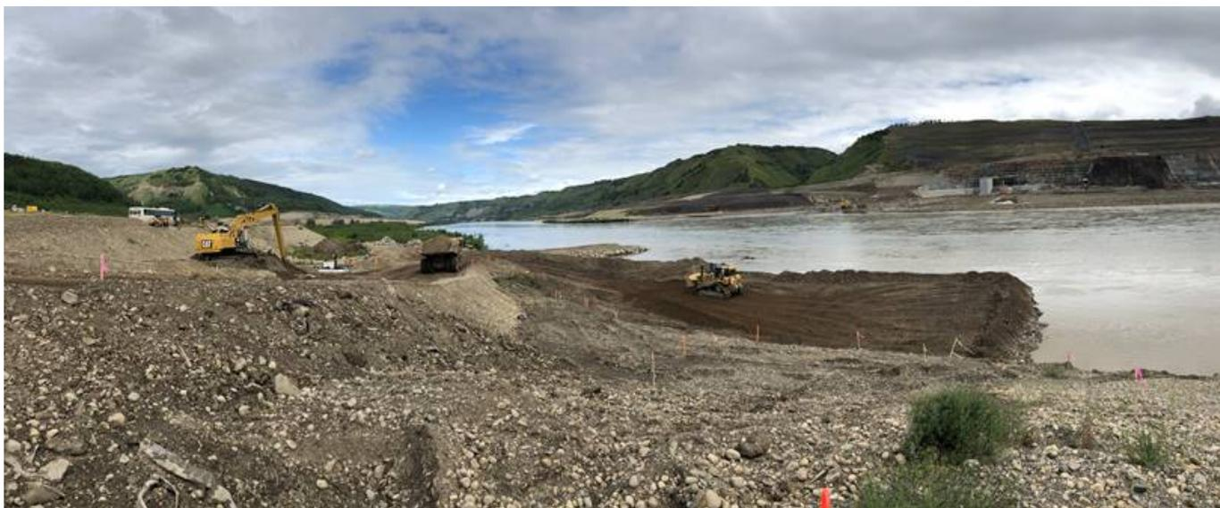
A haul truck (centre) transports material that will be placed on the upstream cofferdam base and spread out by the bulldozer (right). See more project photos in the [image gallery](#).
