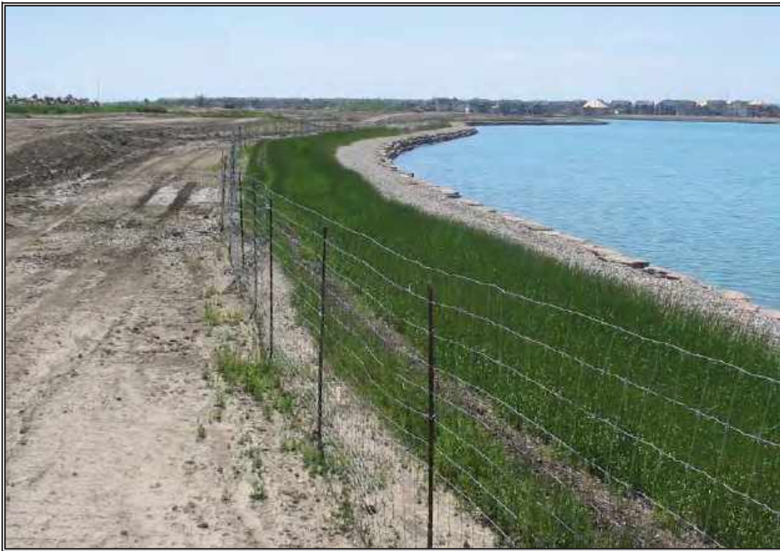
Protection of water body adjacent to a stripped area of land is enhanced with a seeded compost berm and compost blanket (promotes filtering of sediment-laden run-off and provides an erosion-resistant buffer.
