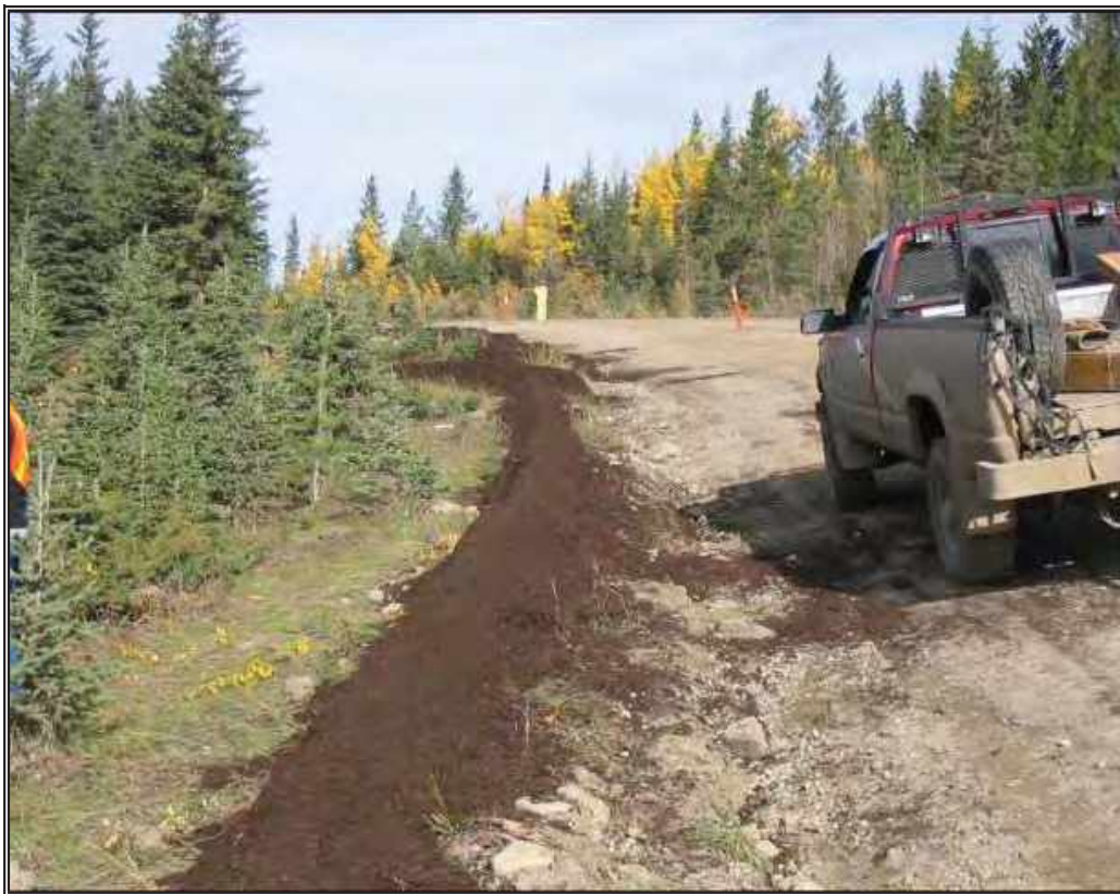
Installation of a compost berm
