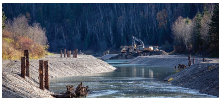
Construction of new downstream channels for fish habitat
