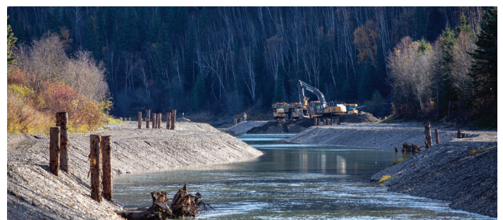
Construction of new downstream channels for fish habitat
