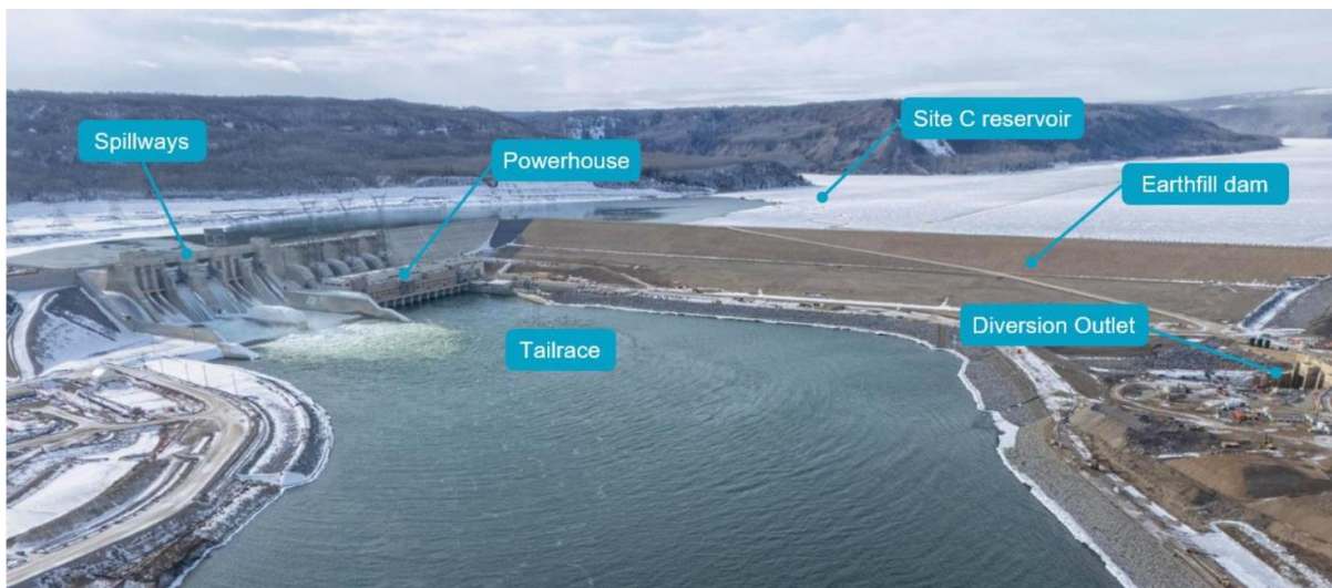
8 Figure 1 Site C - Key Components
