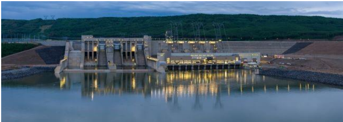
Figure 2 Site C Dam - Spillway (Centre Left), Generating Station (Centre Right) and Transmission Lines (Above the Generating Station).
