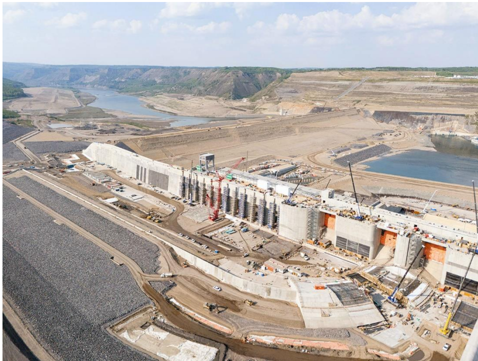
9 Figure 3 Approach Channel, Power Intakes, and 10 Spillway Intake Structures in 11 August 2023
