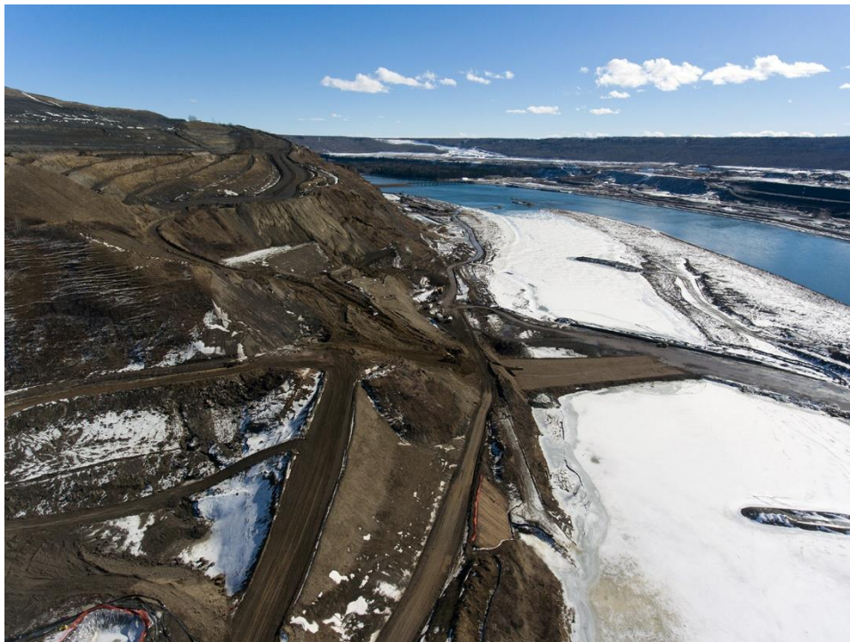
Figure 2 Left Bank Toe Berm Construction in March 2017
