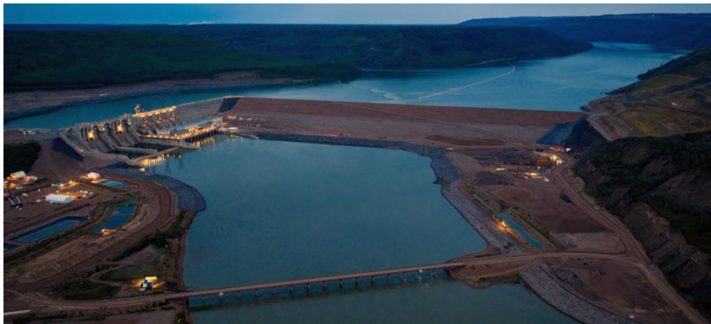
Figure 1 The Site C Dam, Generating Station, and Spillways in August 2025
