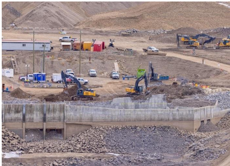
Figure A-8 The removal of the temporary upstream fish passage structure. (April 2025)
