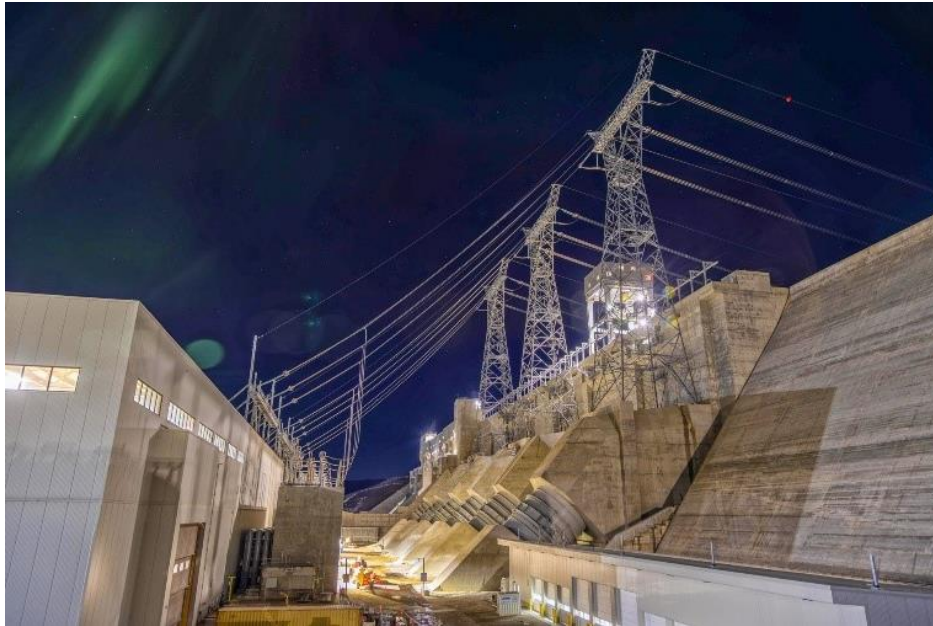
Figure A-1 The back of the powerhouse (left) and the transformer yard, showing the six penstocks and the three transmission lines between the powerhouse and the Site C substation. (April 2025)
