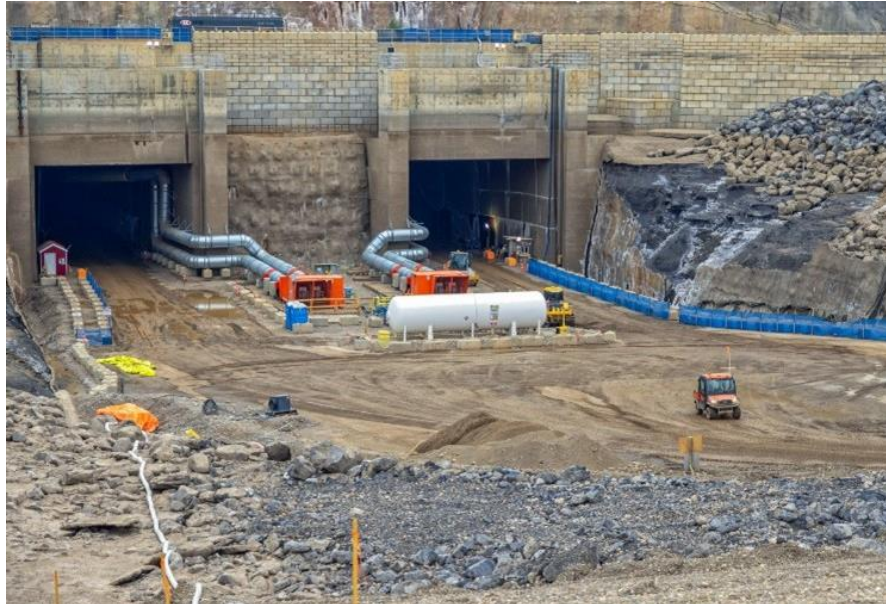
Figure A-7 The dewatered diversion tunnel outlet portals. Temporary ventilation maintains airflow in the tunnels while the backfilling work is underway. (June 2025)
