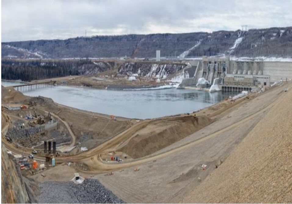
Figure A-4 Photograph looking downstream. In the bottom left of the photo are the north abutment drainage channel and the diversion tunnel outlet. On the right of the photo are the spillways and generating station. (April 2025)
