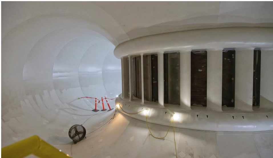
Figure A-15 Inside the unit 6 scroll case. (April 2025)
