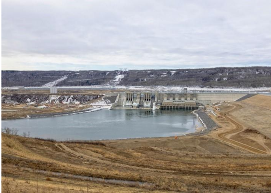
Figure A-2 The downstream side of the spillways and generating station, with the earthfill dam on the right. (April 2025)
