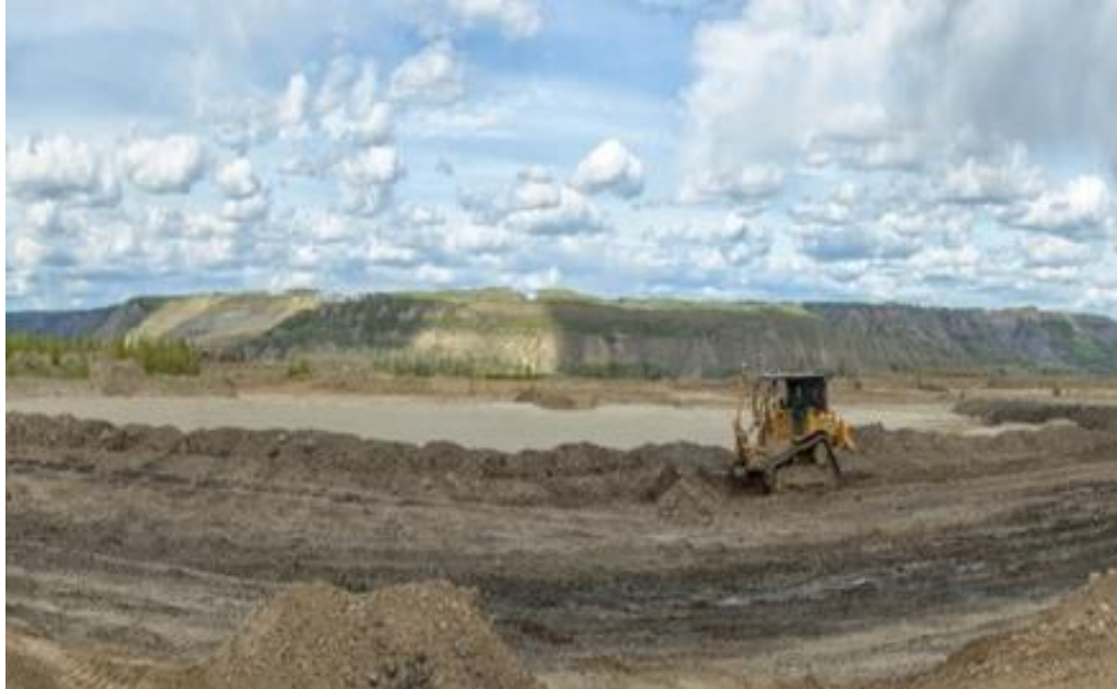
Figure A-17 Re-grading the grassland reclamation area. (May 2025)
