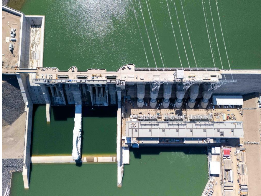
Figure A-6 Photograph looking down on the Site C facility. The spillways are on the left, and the powerhouse is on the right. (April 2025)
