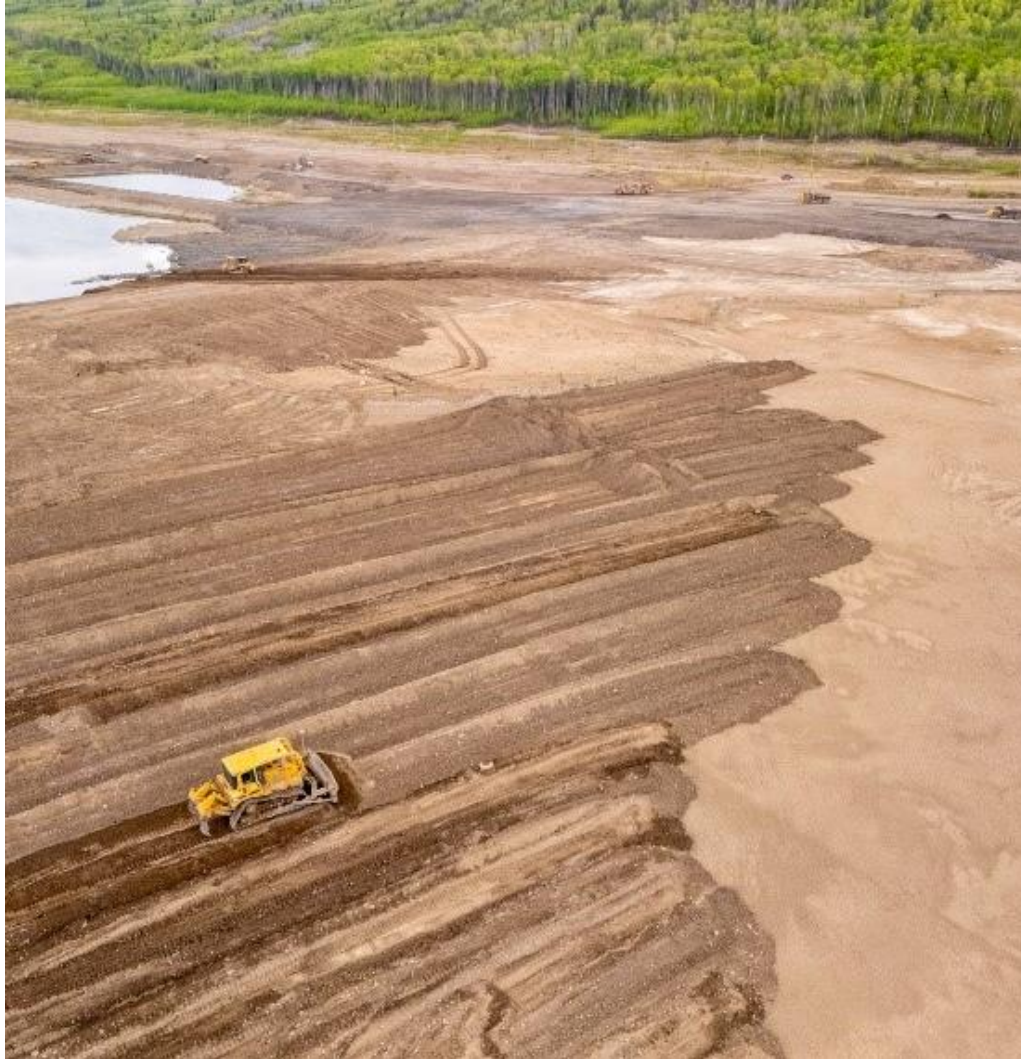
Figure A-16 Re-grading the grassland reclamation area. (May 2025)
