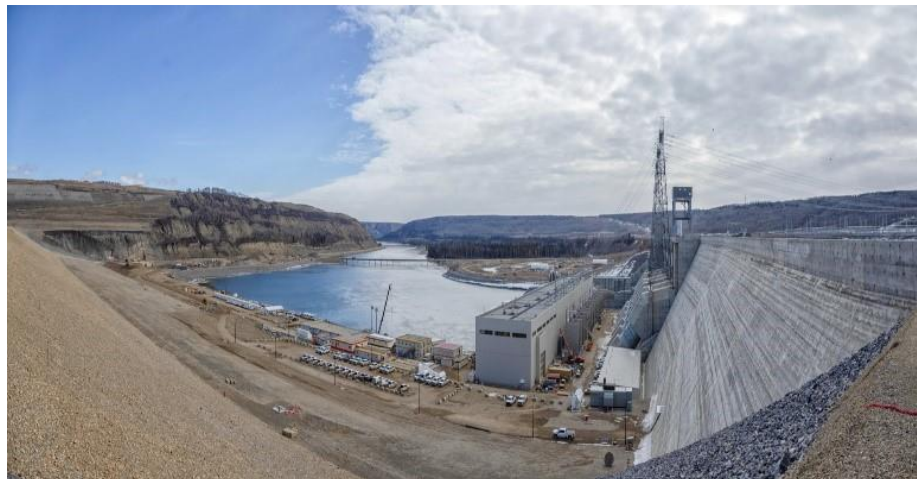
Figure A-3 Downstream view from the dam crest of the concrete buttress wall, showing the transformer yard and powerhouse. (April 2025)
