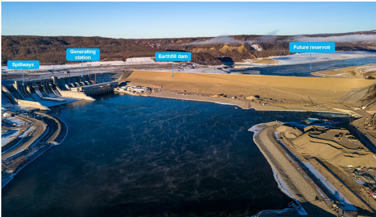
The Site C dam site (as seen in March 2024).
