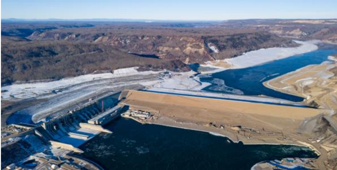
Figure A-5 Looking upstream at the earthfill dam, with the approach channel located behind and to the left of the spillways, penstocks, the powerhouse, and the operations building | February 2024
