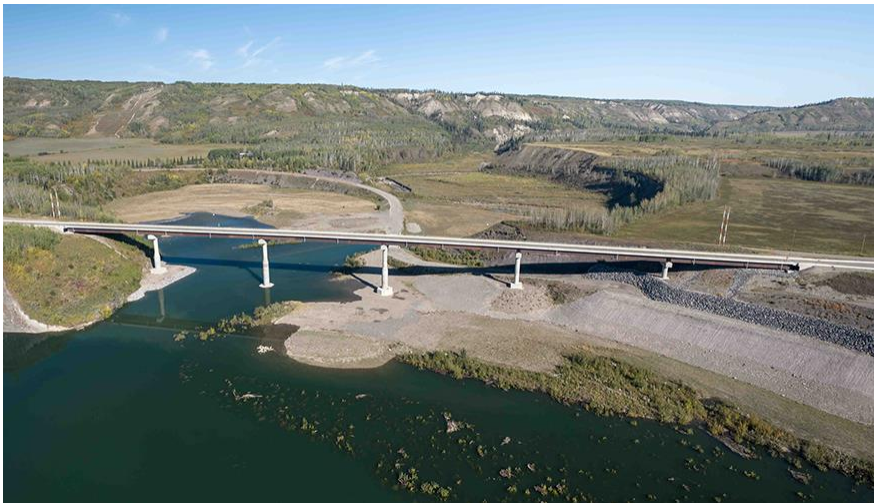
The Farrell Creek bridge on September 12, 2024. See more photos and video of reservoir fill in our gallery.
