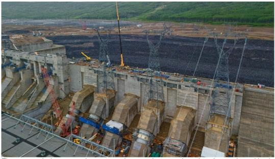
Three transmission towers that connect the powerhouse to the substation are in position in preparation for first power later this year. See more construction photos in our gallery.
