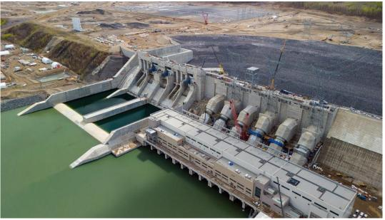
When the Site C dam is fully operational, water will flow down the approach channel, through the intakes, and down the six penstocks to the generating station below. See more construction photos in our gallery.
