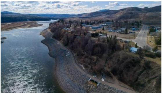
The Hudson's Hope berm will reinforce the shoreline and protect it from potential erosion once the Site C reservoir is filled. See more construction photos in our gallery.
