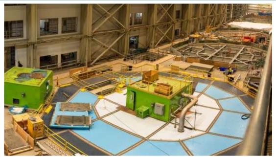
Inside the powerhouse, turbine unit 1 nears completion with brush housing and floor panels installed. <u>See more construction photos in our gallery.</u>
