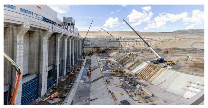
Workers place formwork and reinforcing steel on the erosion slabs in the Site C tailrace. <u>See more construction</u> photos in our gallery.
