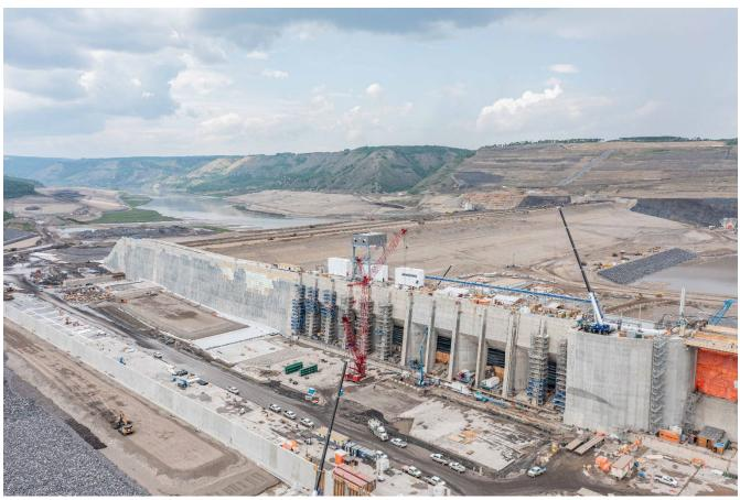
When the Site C reservoir is filled, water will flow down the approach channel to the intakes, which lead to the powerhouse. In the background, construction of the earthfill dam continues. See more photos in <u>our gallery</u>.
