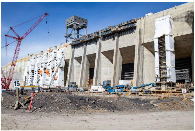
We recently completed concrete work for the intakes. When the Site C reservoir is filled and the dam is operating, the intakes will funnel water into the penstocks, which lead to the turbines in the powerhouse. See more photos in <u>our gallery</u>.
