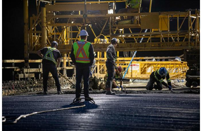
Crews work overnight to complete a concrete pour on the Lynx Creek Bridge deck, as part of the Highway 29 realignment. See more photos in the <u>image gallery</u>.
