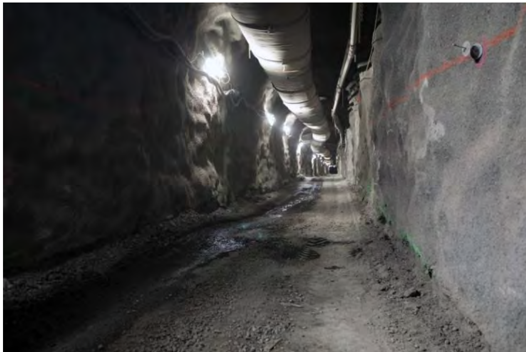
Figure A-6 Drainage Tunnel on the Right Bank (March 2018)
