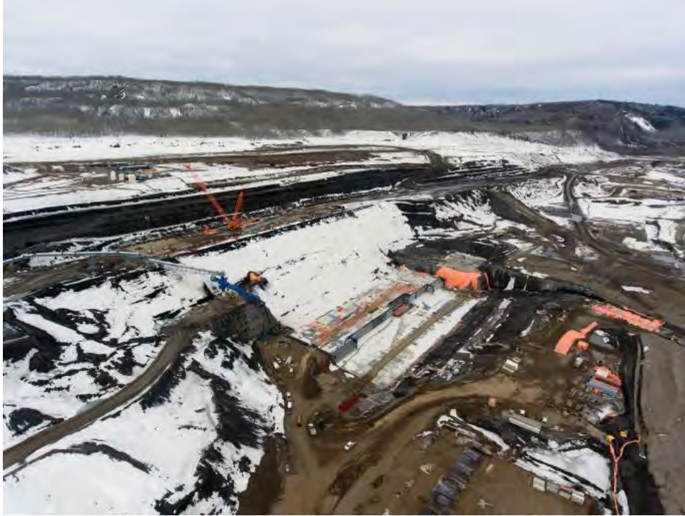
Figure A-9 Right Bank Roller-Compacted Concrete Area (April 2018)
