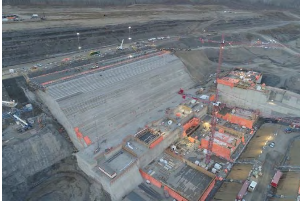
Figure A-27 Completed Powerhouse Buttress on the Right Bank (October 2018)
