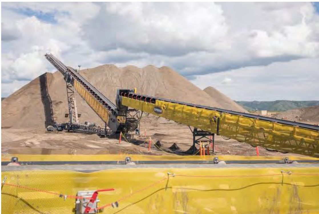
Figure A-14 Right Bank Phase 2 Crusher (June 2018)
