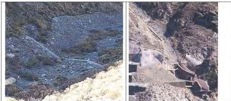
Reno mattresses lining creek on Cairnmuir landslide (New Zealand).
