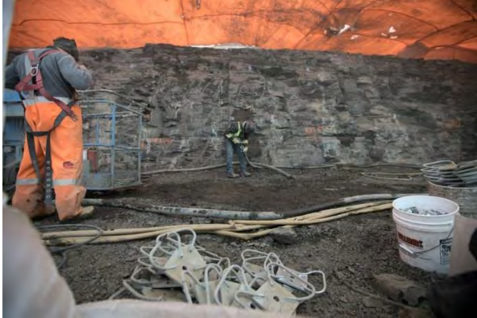
Figure A-11 Left Bank Shotcrete Placement for the Inlet Portal (April 2018)
