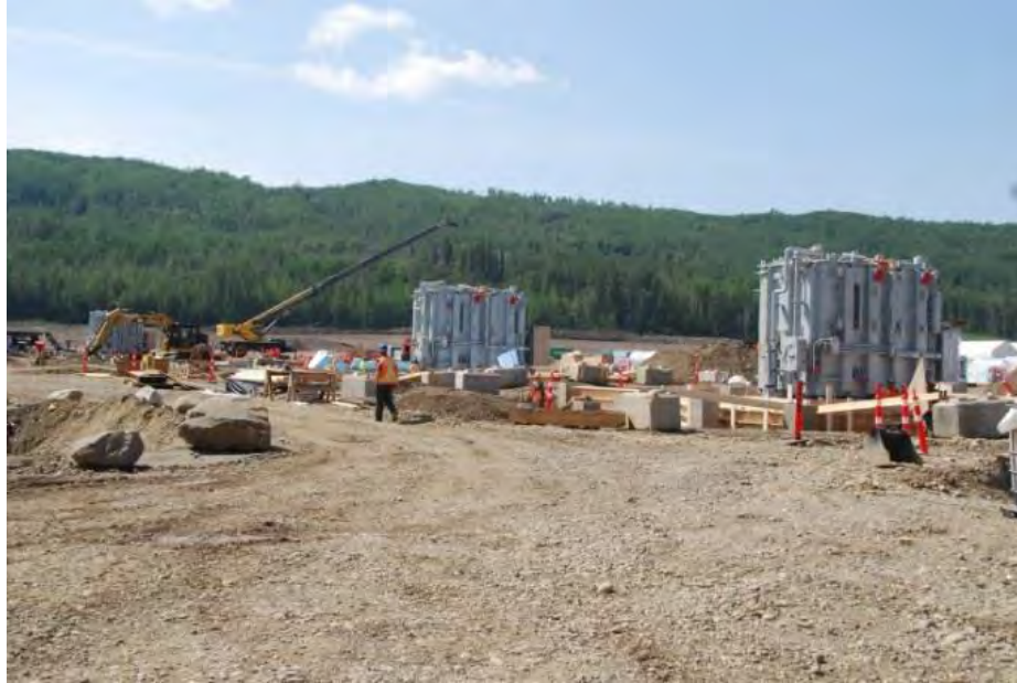
Figure A-21 Transformer Assembly at the Site C Substation Site (August 2018)
