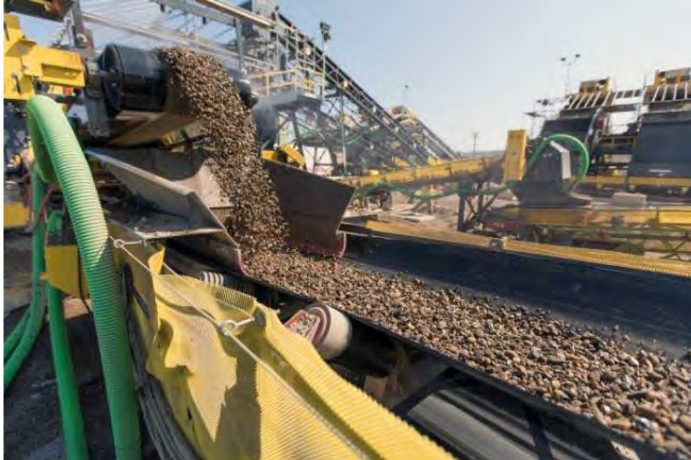
Figure A-17 Right Bank Phase 2 Crusher Plant (July 2018)
