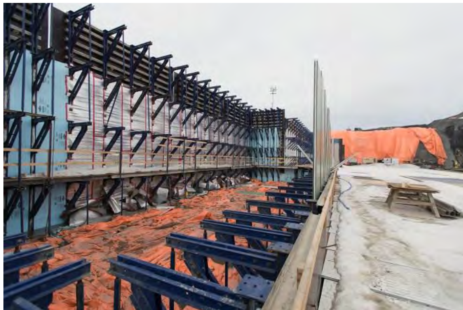
Figure A-8 Right Bank Insulation Placement on the Face of the Roller-Compacted Concrete (April 2018)
