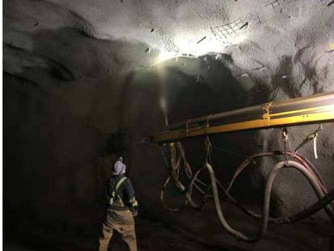
Figure A-23 Shotcrete Application in the Right Bank Drainage Tunnel (August 2018)
