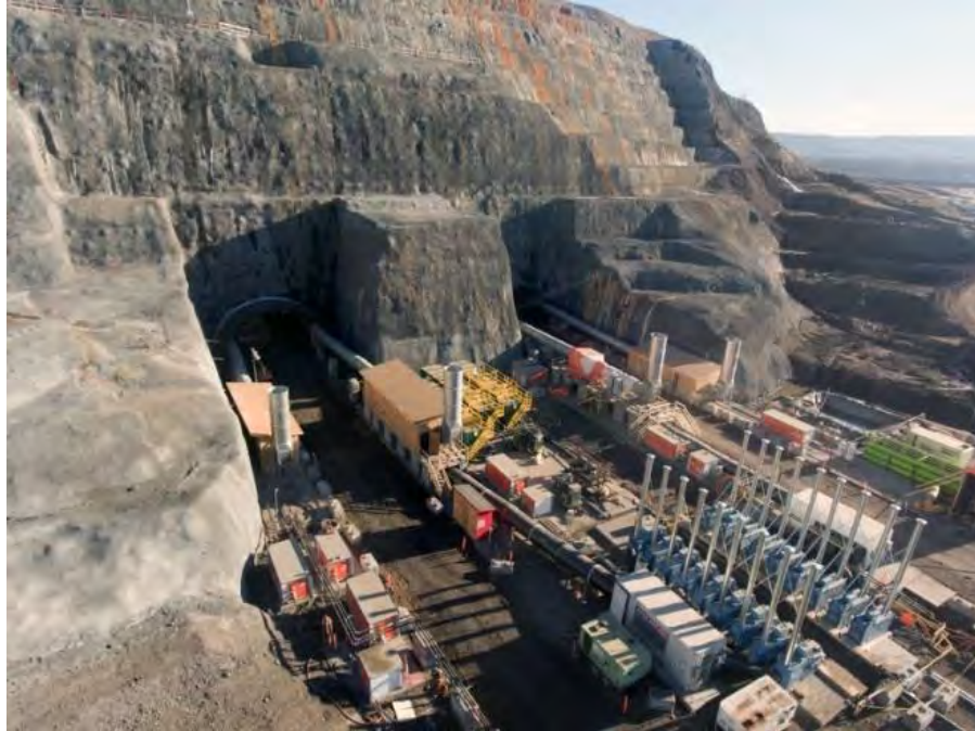
Figure A-31 Excavation of Diversion Tunnels on the Left Bank (October 2018)
