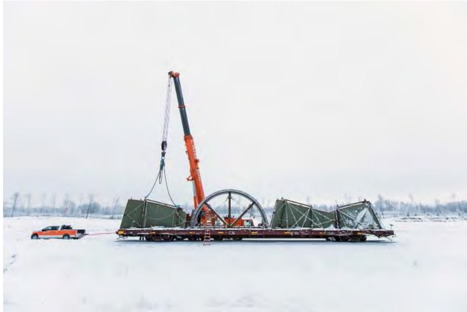
Figure A-1 The Turbines and Generators Contractor Delivering Equipment to their Work Area (January 2018)
