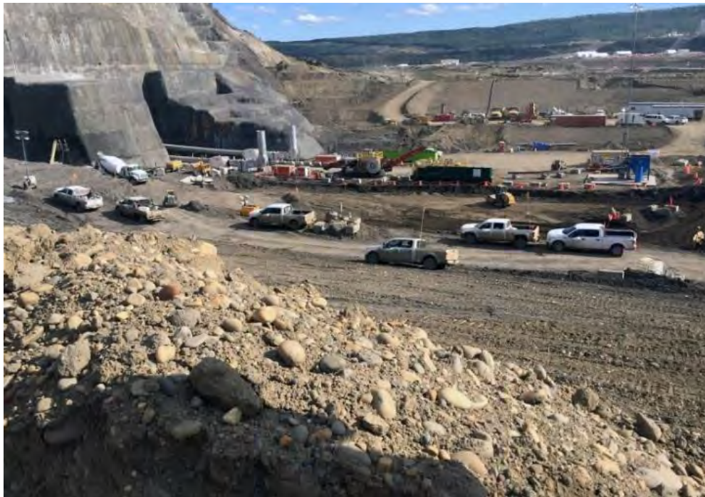
Figure A-26 Work on the Diversion Tunnel Inlet Portal (September 2018)
