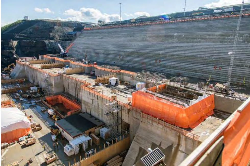
Figure A-25 Powerhouse Construction Area (September 2018)
