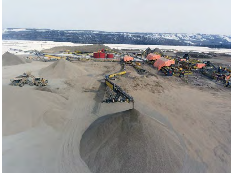
Figure A-7 Right Bank Crusher Plant 2 and Aggregate Stock Piles (April 2018)
