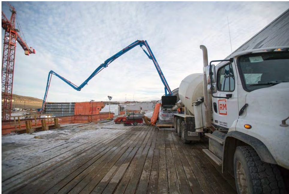
Figure A-36 Concrete Being Pumped into a Coupling Chamber at the Powerhouse (December 2018)
