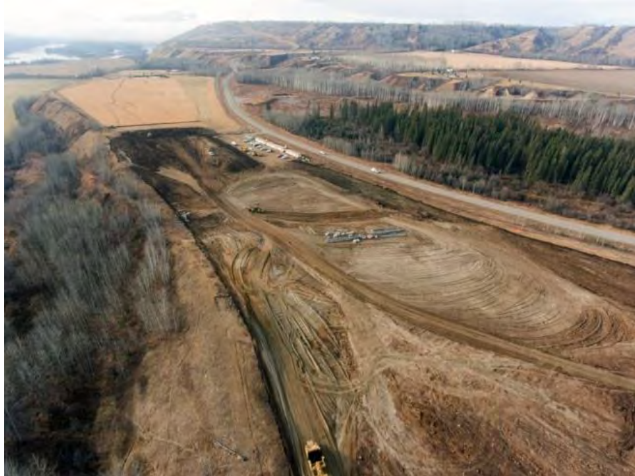
Figure A-29 Laydown Area for Highway 29 Cache Creek West Construction (October 2018)
