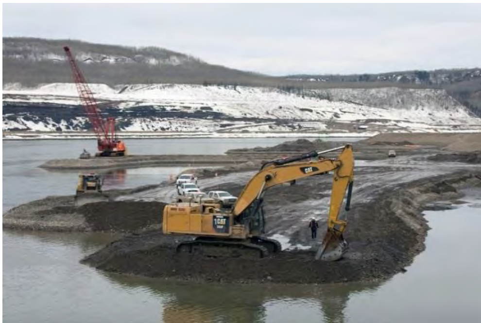
Figure A-10 In-River Works – Dredging (April 2018)
