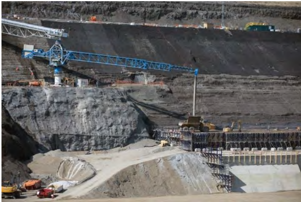
Figure A-18 Concrete Placement for the Right Bank Powerhouse Buttrass (July 2018)
