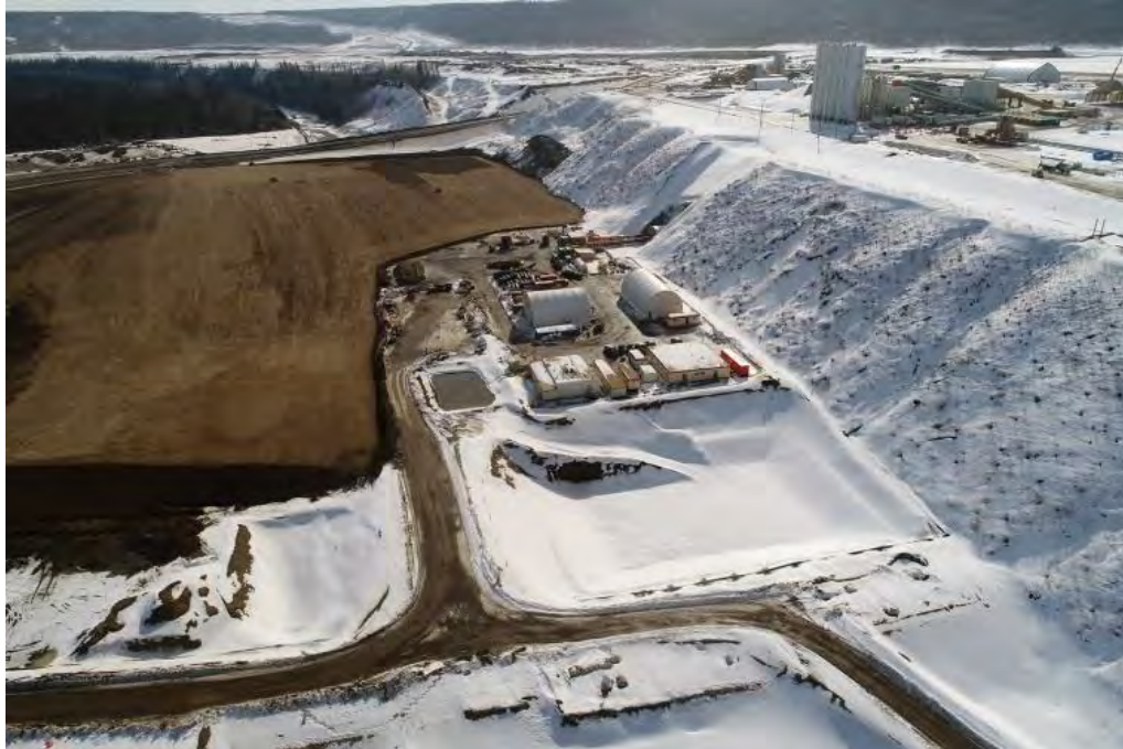
Figure A-5 Aerial View of the Drainage Tunnel on the Right Bank (March 2018)
