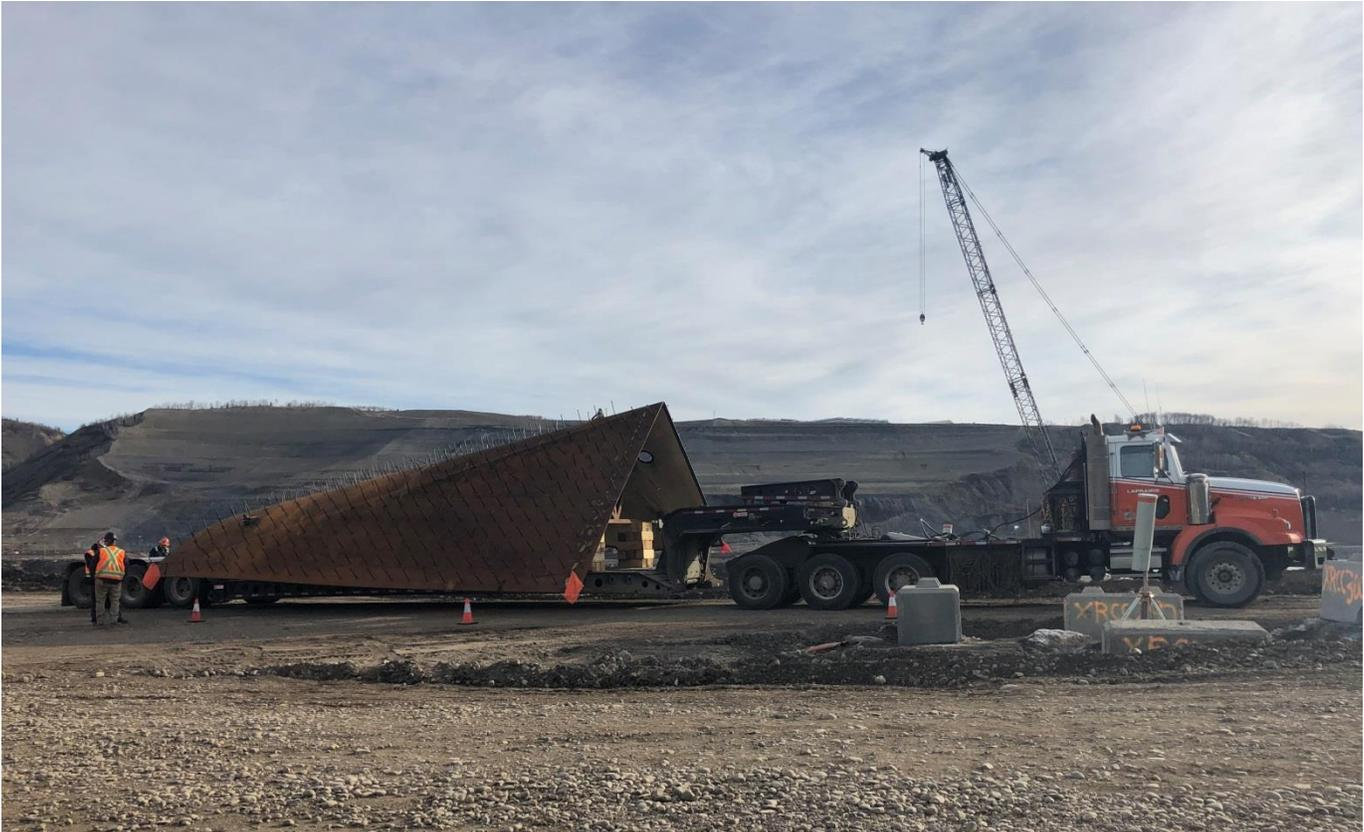
Photo: Large sections of penstocks are being delivered to site, along Old Fort Road.
