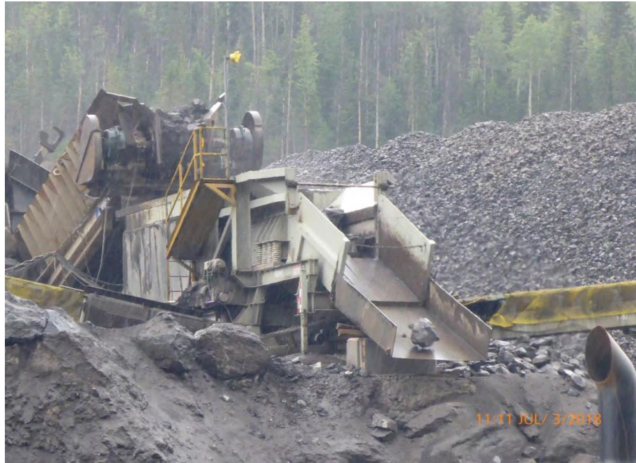
Figure A-1 West Pine Quarry Facing North. Photo taken July 3, 2018.
