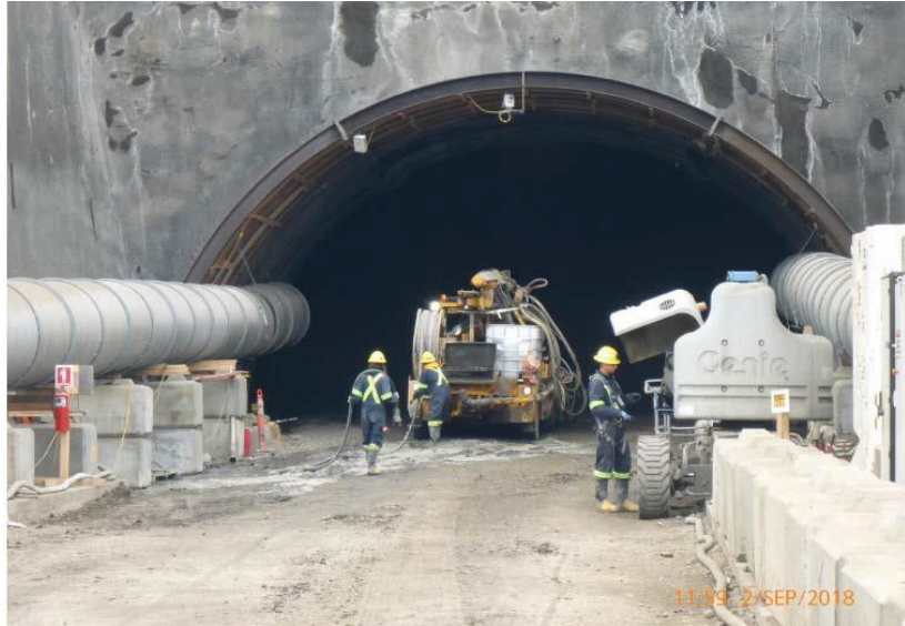
Figure A-7 Shotcrete Work in Tunnel 1. Photo taken September 2, 2018.
