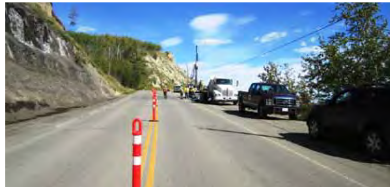
Highway 29: Geotechnical Investigations
