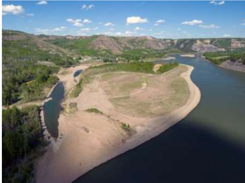
Figure A-8 One of the many fish habitat offsets constructed as part of the Site C Project. Reclamation planting is complete at this location | May 2024
