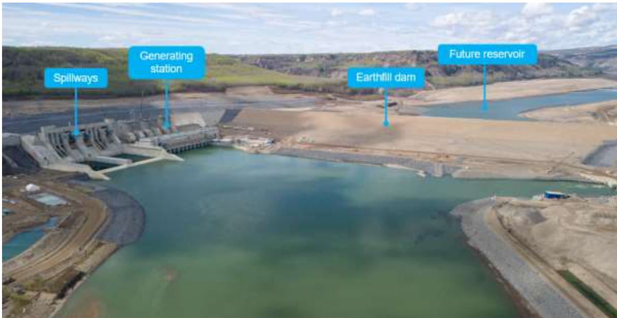
The Site C dam site (as seen in May 2024).
