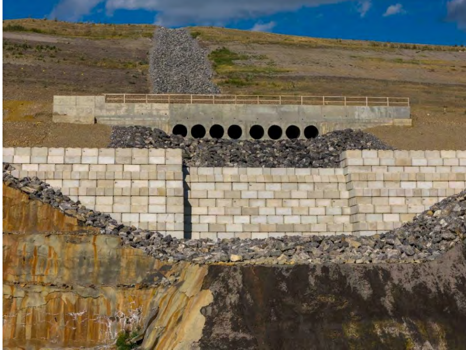
Figure A-6 Completed drainage management structure
