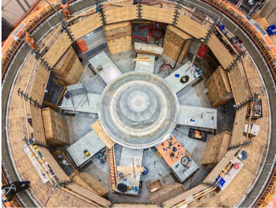
Figure A-8 Brazing stator windings on turbine unit 6
