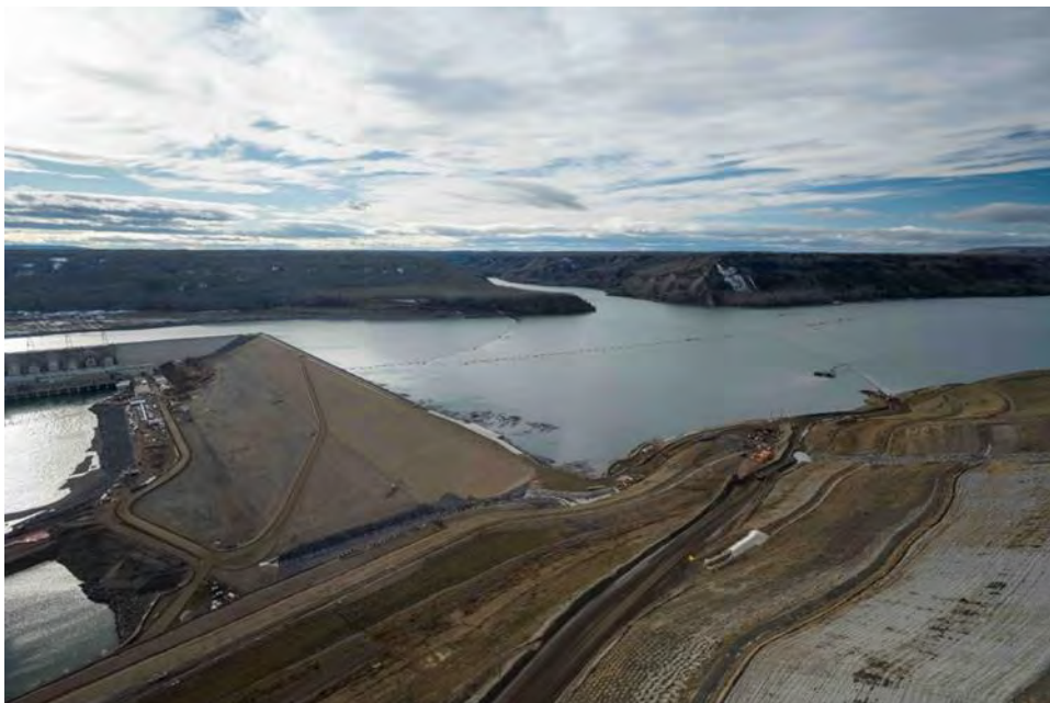
Figure A-13 The Site C reservoir at the dam, with the Moberly River at centre
