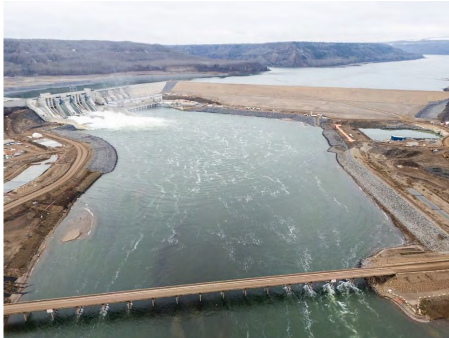
Figure A-10 The Site C dam and generating station in October 2024
