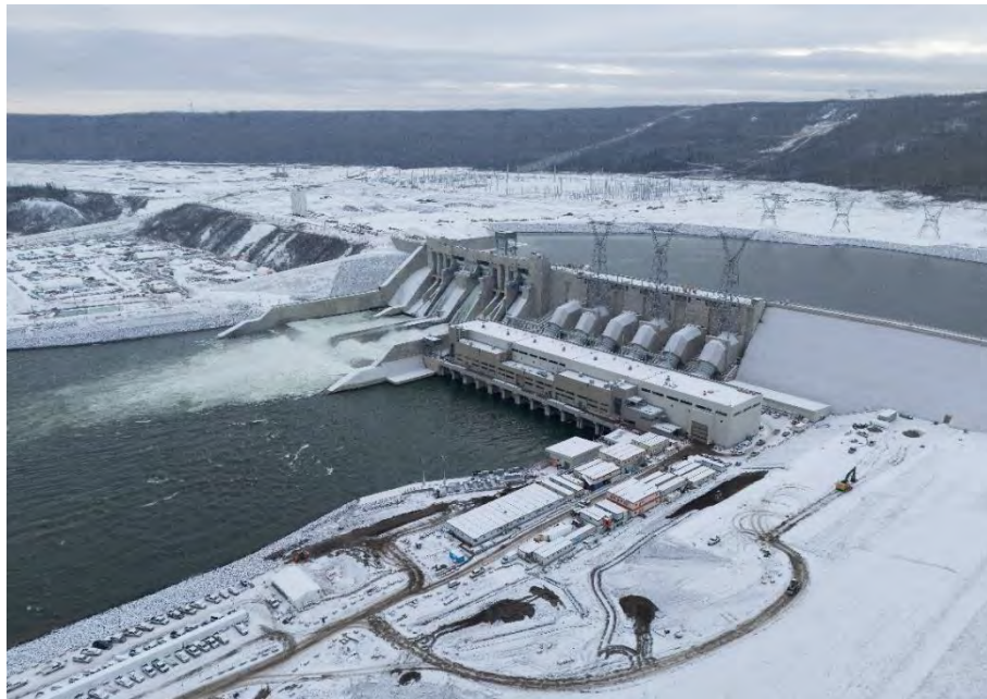
Figure A-15 Unit 1 is generating power from Site C and water is passed through the spillways to maintain downstream flows
