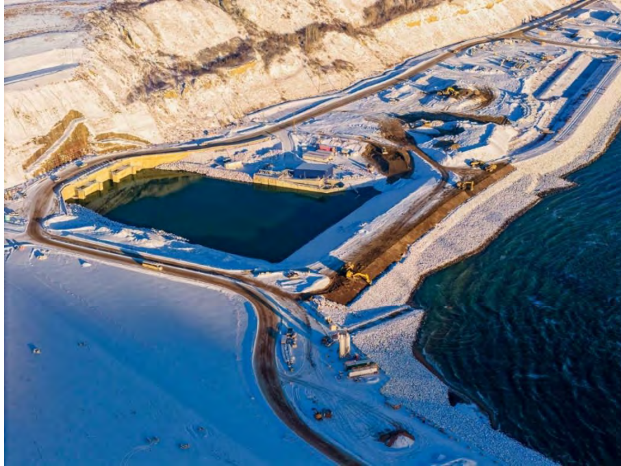
Figure A-14 A cofferdam nears completion at the diversion outlet portals
