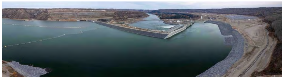
Figure A-4 The Site C reservoir at the dam and approach channel
