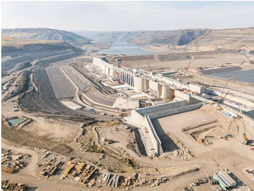
**Figure A-10** Riprap is one of the many protective layers in the approach channel where water will flow from the reservoir into the powerhouse and spillways | September 2023
