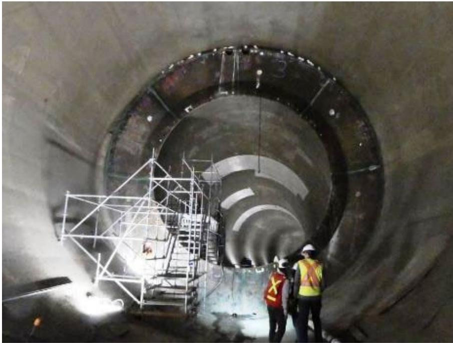
Figure 4.11 – Diversion Tunnel Orifice
