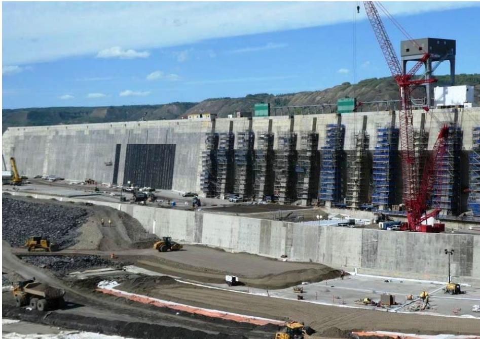
Figure 4.13 – Intakes and RCC Tailrace Wall
