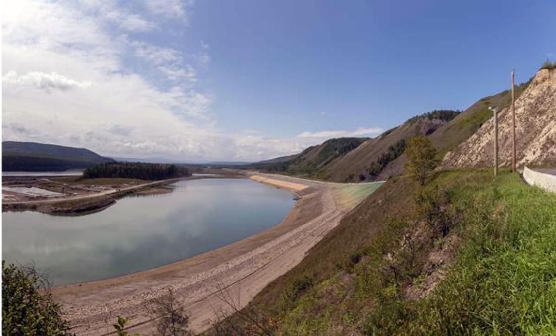
**Figure A-6** Construction continues on the approach channel that directs the flows from the Peace River to the powerhouse and spillways | August 2023
