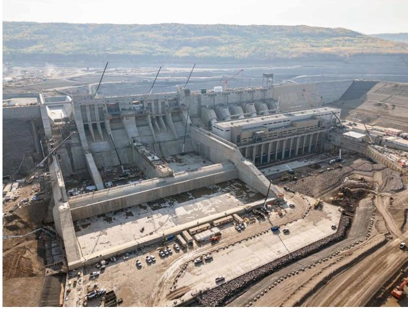
**Figure A-8** Crews are finishing concrete placement for the tailrace erosion protection slabs below the powerhouse. Workers are also excavating the interior of the right bank cofferdam and placing riprap | September 2023
