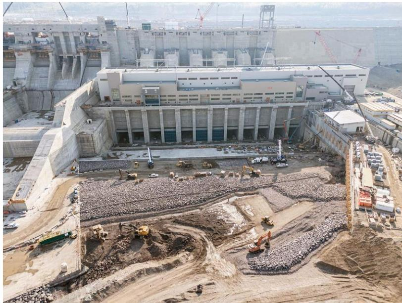
**Figure A-9** When the Site C reservoir is filled, water will flow down the approach channel and enter the powerhouse through the intakes, or the entrances to the spillways | September 2023
