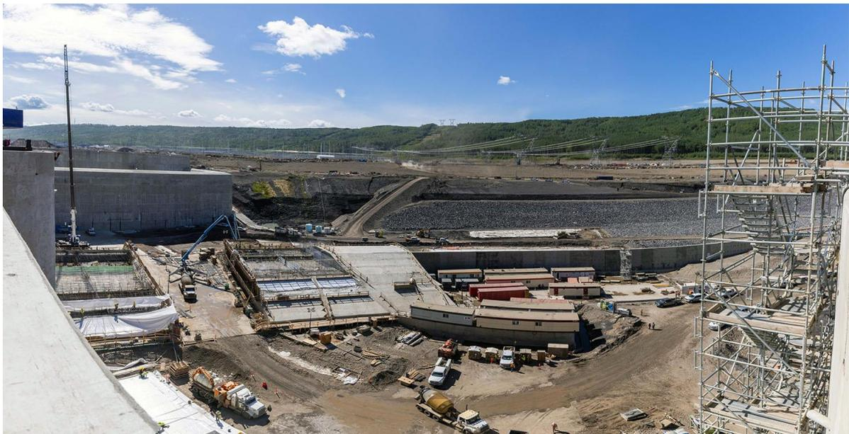
**Figure A-7** In the future, water will go through six penstocks into the powerhouse (on right side of picture), then exit through the tailrace. The spillways on the left will safely pass flows from the reservoir | September 2023
