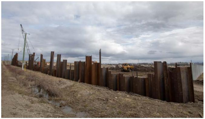
Photo: We're building a reinforced pile wall as we excavate for the conveyor system, which will carry materials from the 85th Avenue Industrial Lands to the dam site. We will cut each pile to the same height once they've been driven to the required depth.
