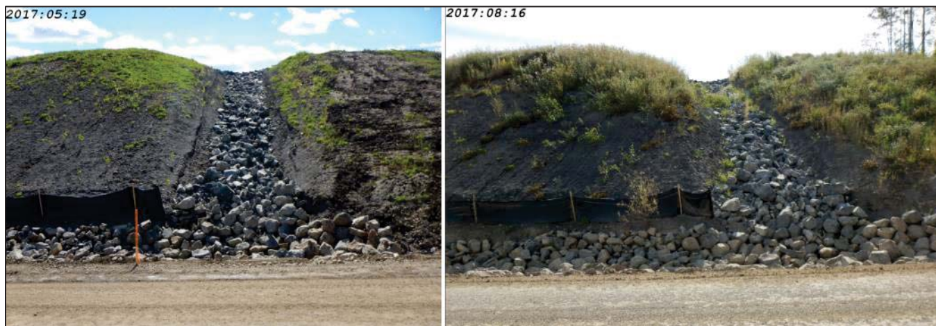
Photo 3: Comparison of vegetation growth at the Blind Corner upper chimney ditch from May 2017 (left) and August 2017 (right)
