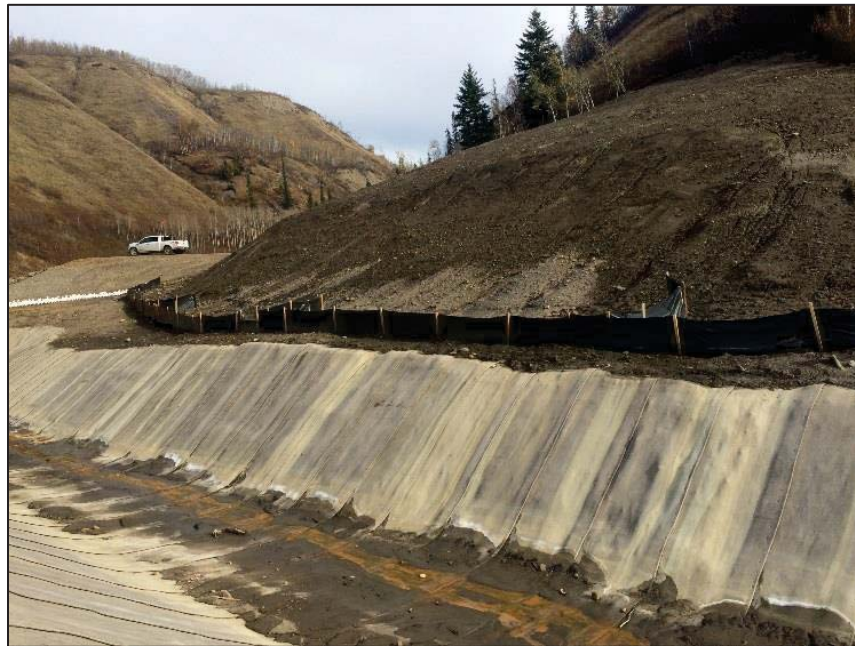
Photo 2: At upper reach of Garbage Creek Diversion ditch, covered PAG slope with NAG Material
