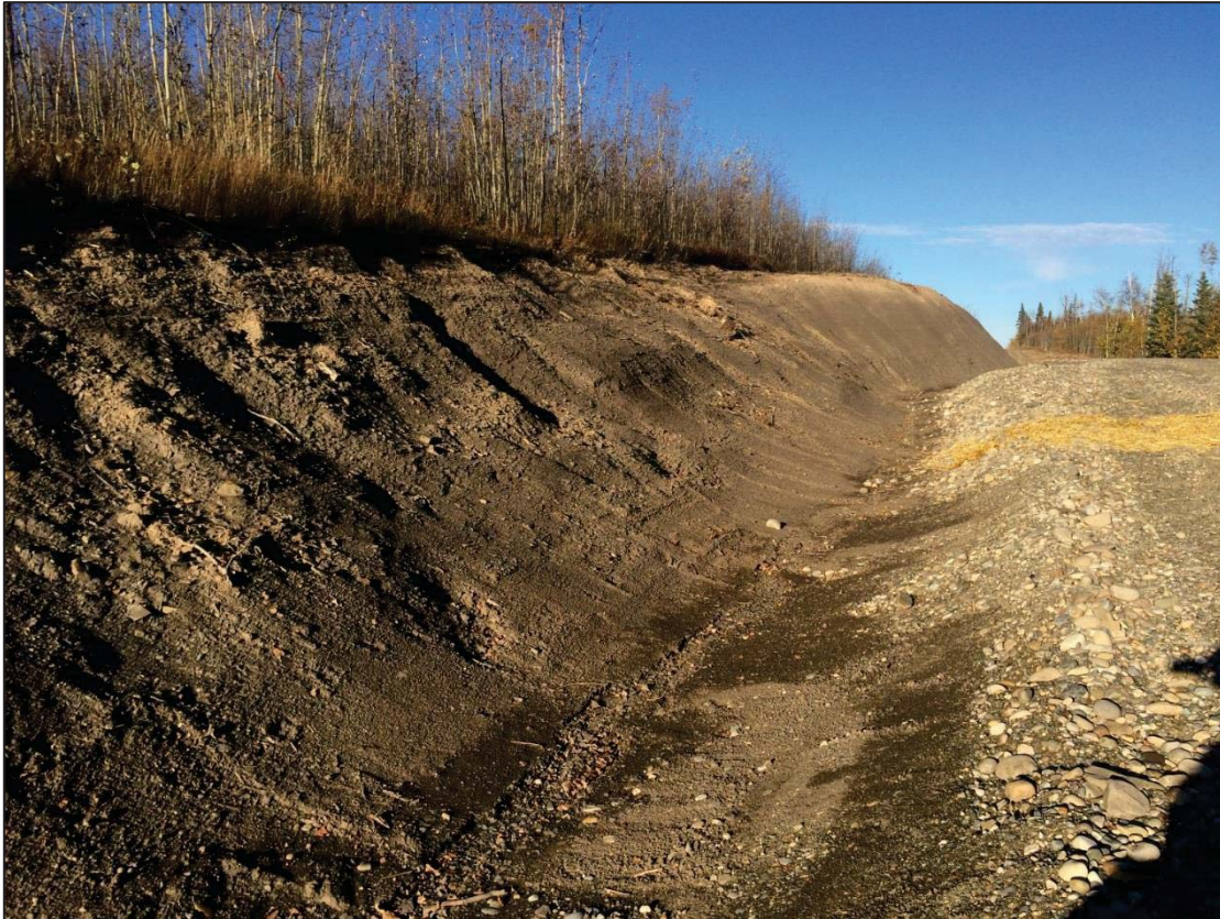
Photo 4: Shale Exposure during Trapper Main upgrade at approximate Chainage 6+500
