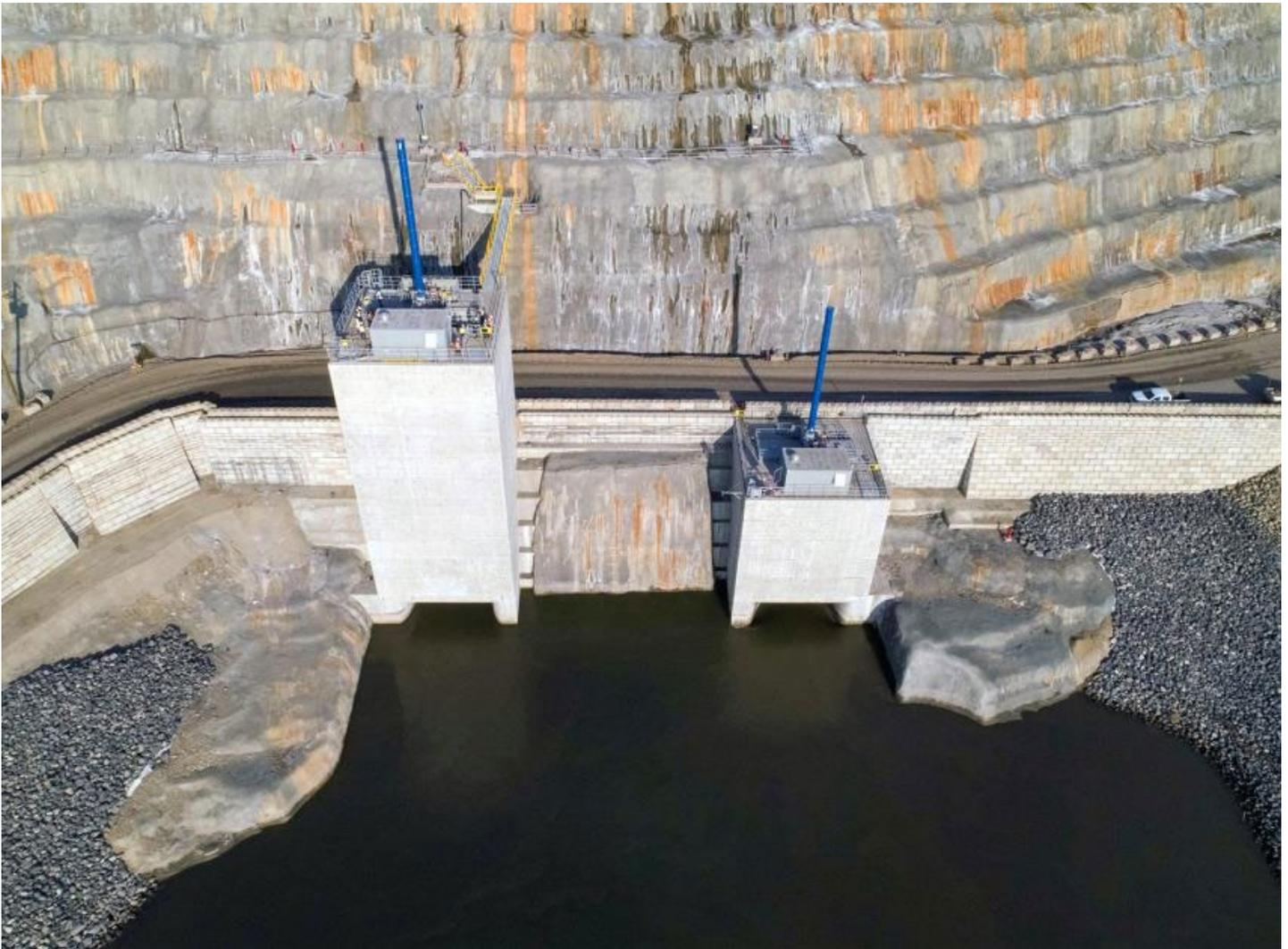
**Photo 5.** Final rip rap is placed on the rockfill berm (center) to close the Peace River on October 3, 2020 (looking downstream).
