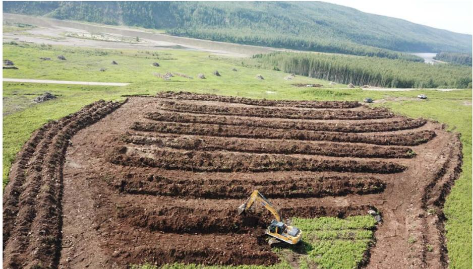
*During archaeology site soil stripping, soil is piled in rows to enable inspection by archaeologists prior to relocation away from the construction site.*
