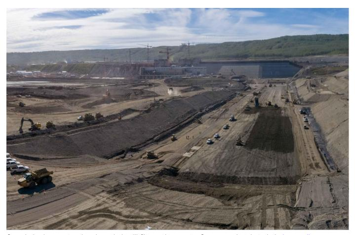
Crews in the dam core trench are busy placing till, filters and aggregates. See more project photos in the image gallery.
