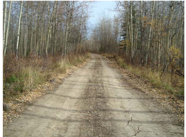
Typical south bank access road
