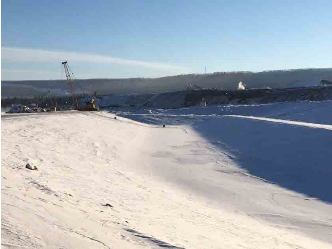
Photo 1. Stormwater Management Settling Pond
