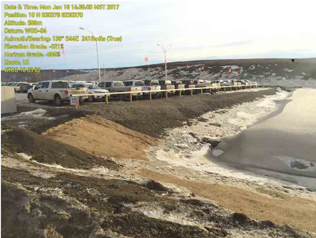
Photo 2. Stormwater Drainage Ditch
