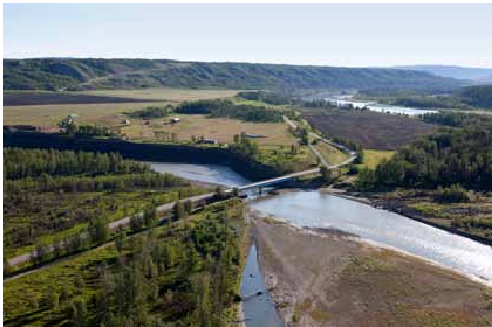
Highway 29 at Halfway River
