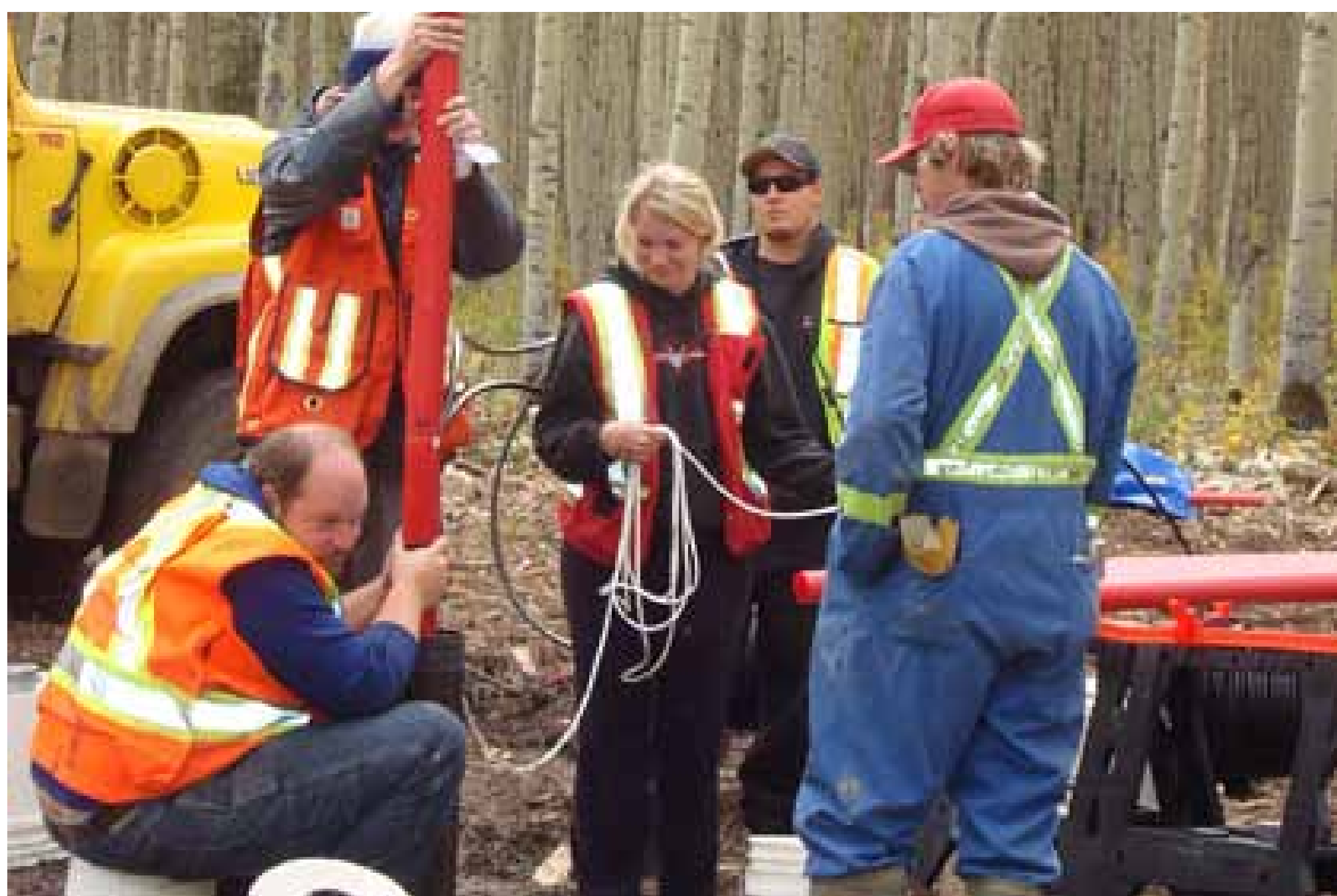
Installing geotechnical instrumentation
