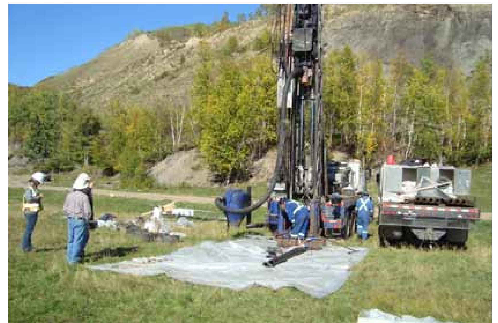
Decker drilling at the proposed dam site
